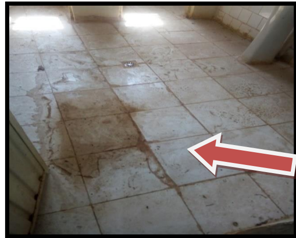
Figure 4.2:- Defective Floor finishes in main entrance Figure 4. 3 :- Defective Floor finishes in Toilet & Shower room
