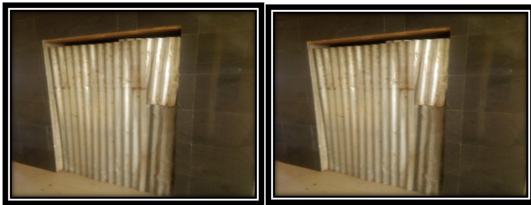
Figure 4.17: the contractors not yet fix the lift machine
