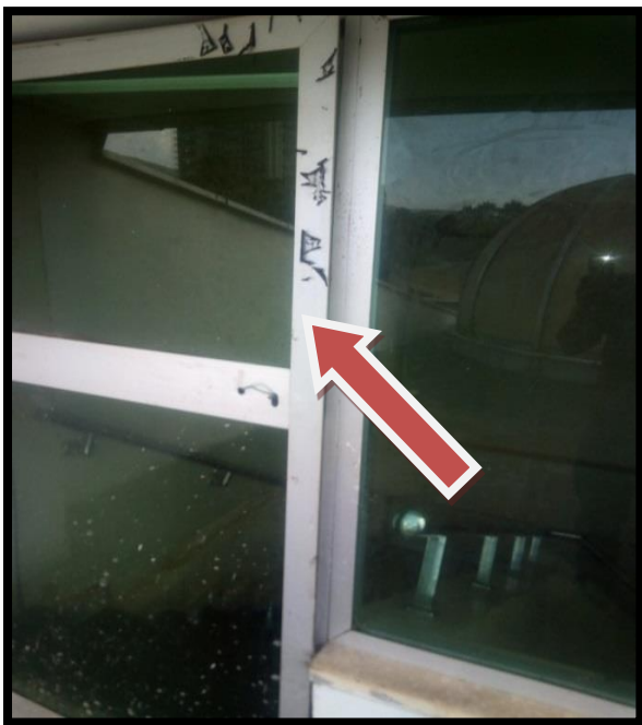
Figure 4.7:- missing of Handling & key
