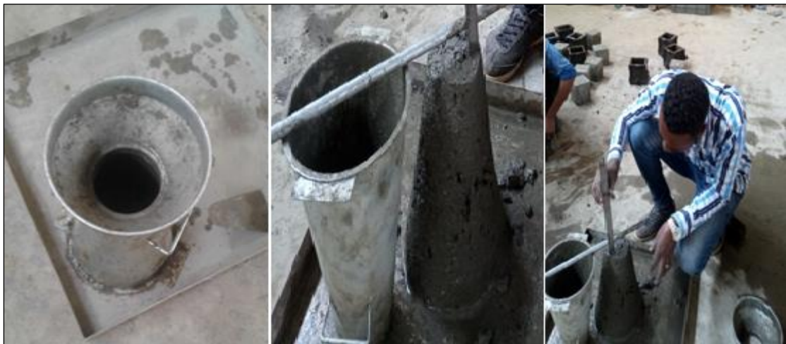
Figure 3.8: Slump Test Procedures
