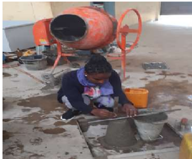
Figure 4.6: Checking of workability of concrete by slump test
