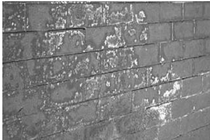
Figure 2.3 Efflorescence
