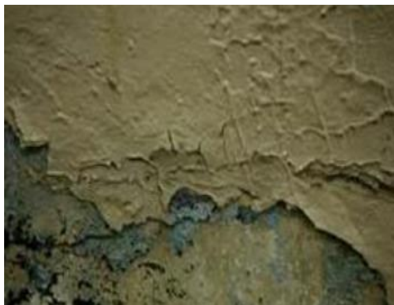
Figure 2.2 Peeling paint
