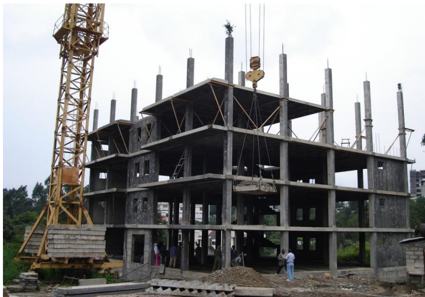
Figure 4.3: Precast concrete building construction
