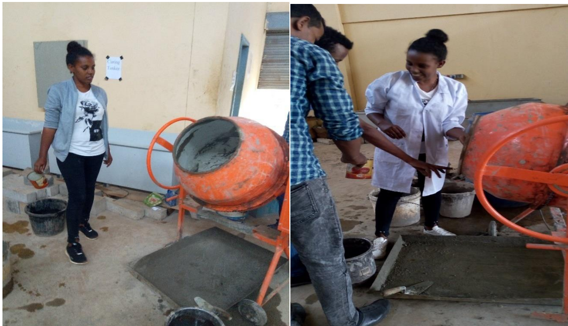
Figure 12 Concrete Mixing Process
