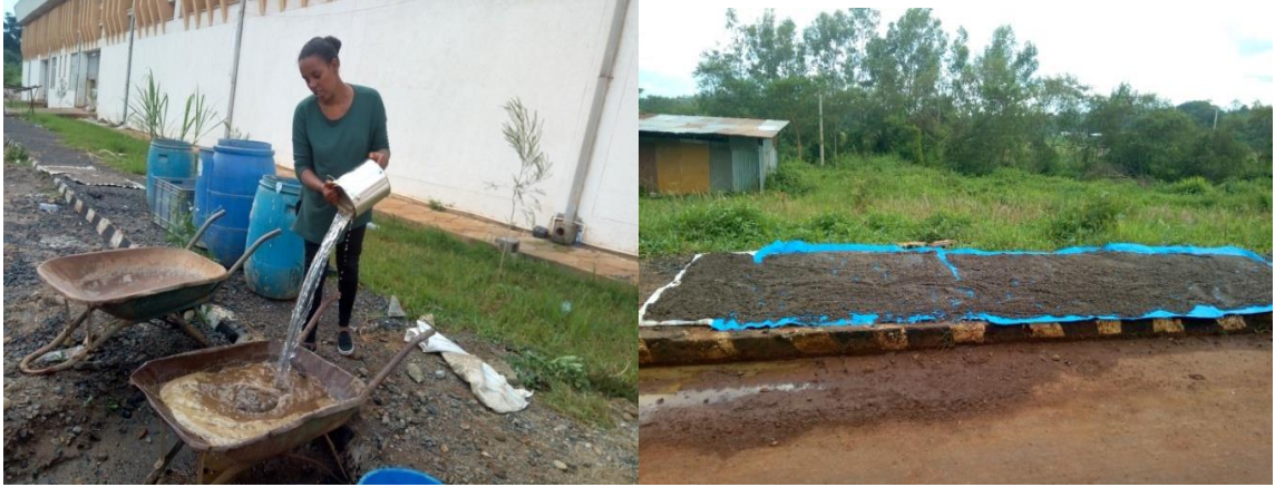
Figure 3. 5 Washing of Sand to make free from silt & clay
