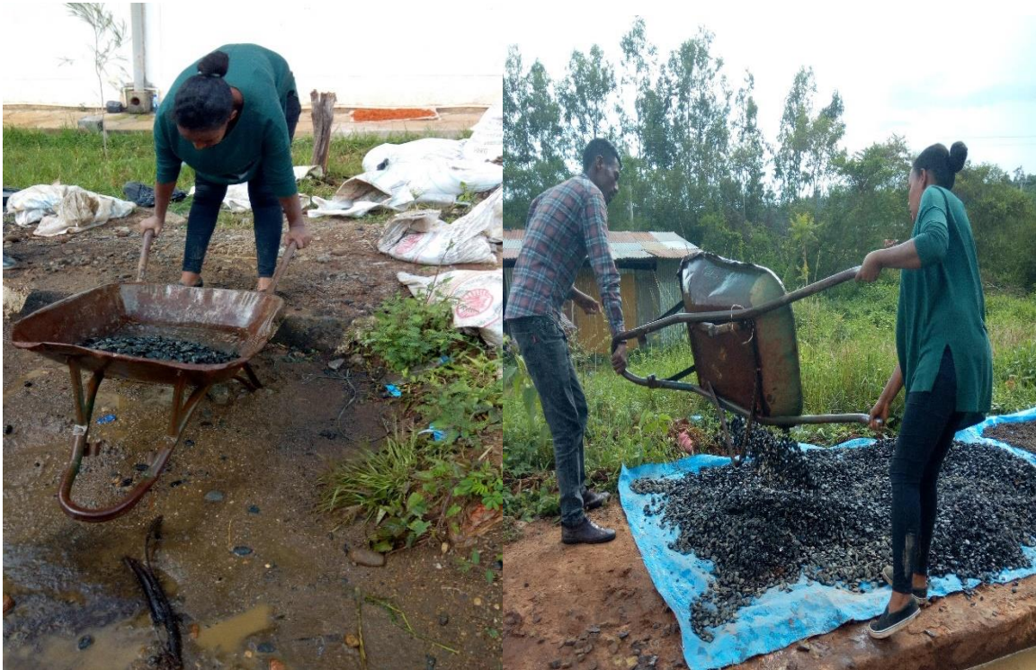
Figure 7 washing of coarse aggregate to make free of clay lump
