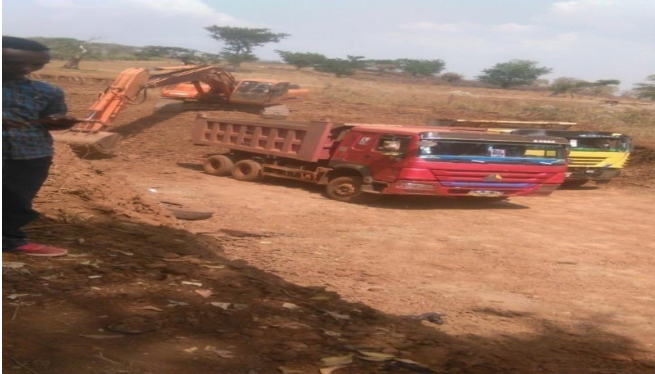
Figure 24 Ongoing project in the study area
