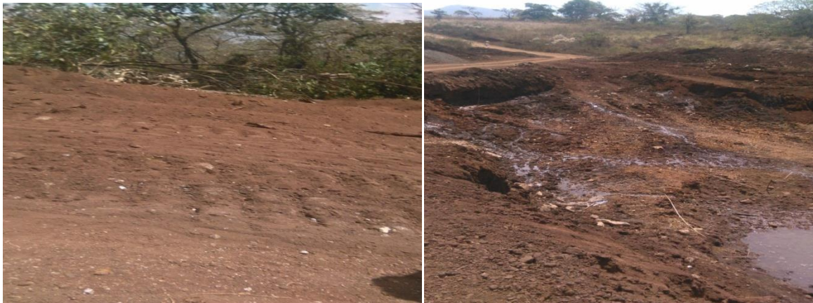
Figure 23 forest land areas opened for new road construction
