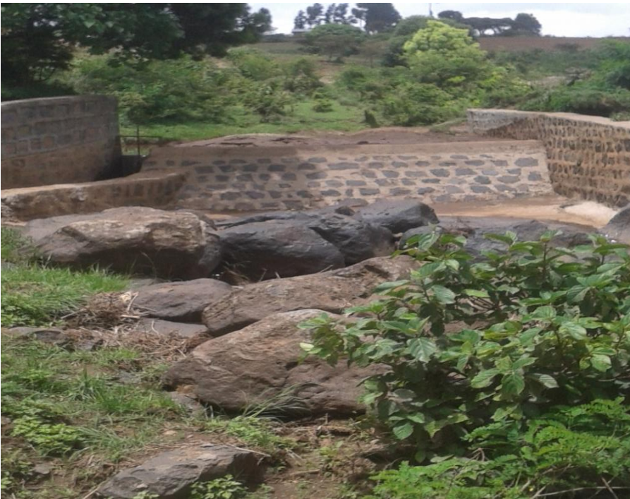
Appendix Figure 7. Diversion weir
