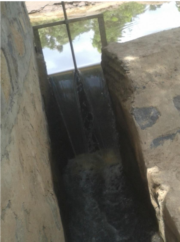
Appendix Figure 4. Intake Gate at Diversion Weir
