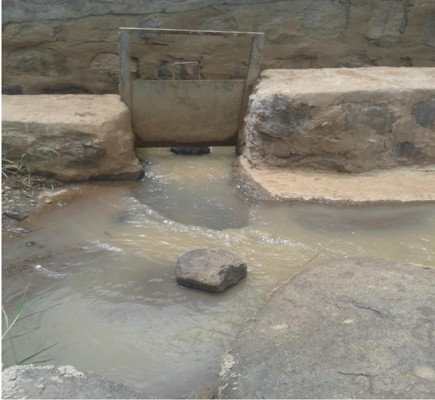
Appendix Figure 6. Sluice gate on main canal
