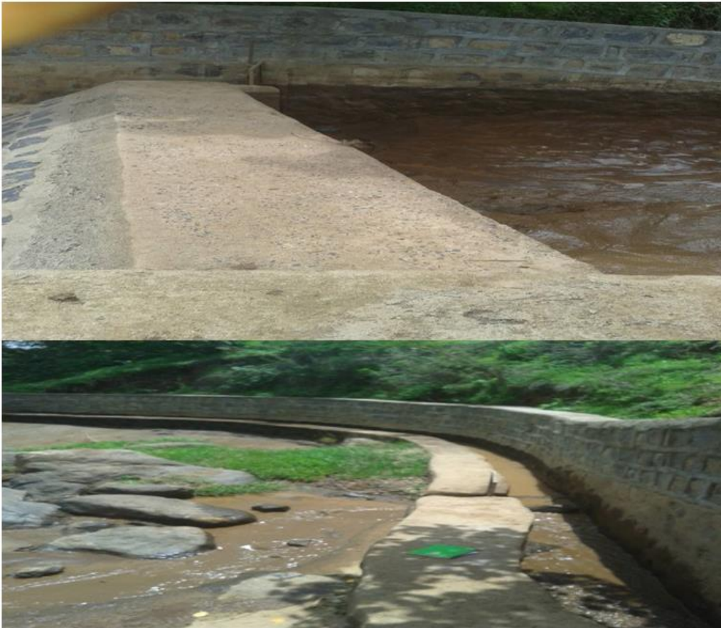
Figure 4.1 Diversion weir and main canal structure of the study site.
