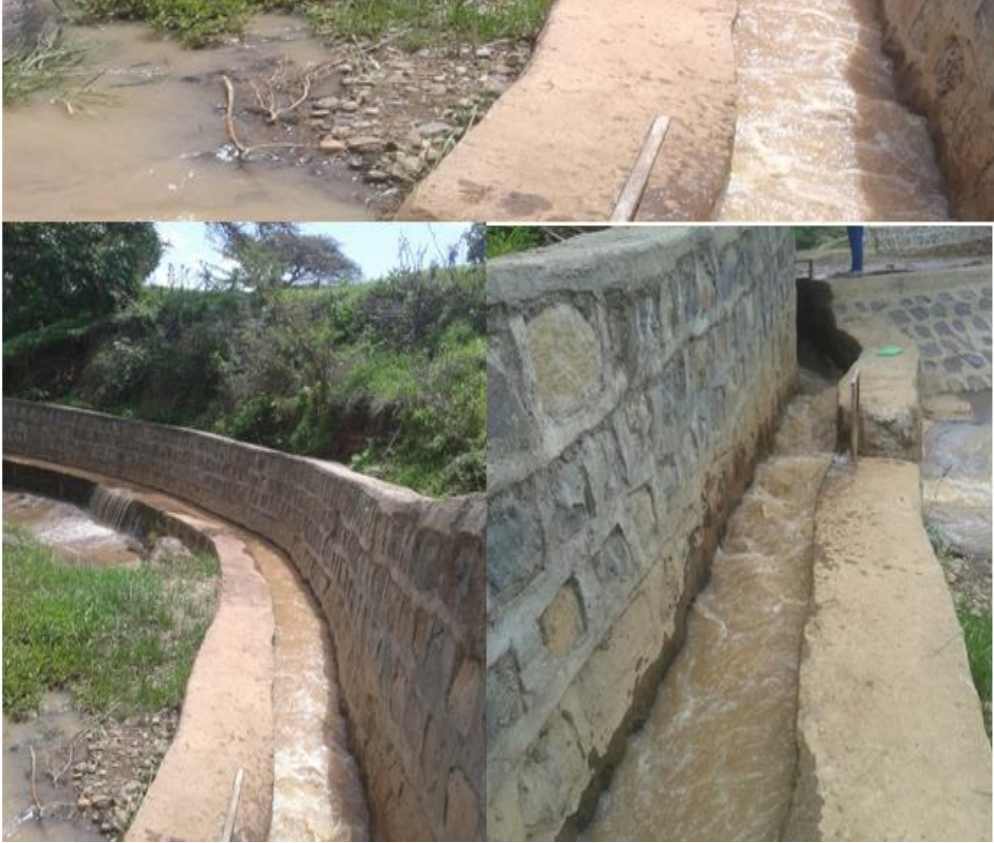
Appendix Figure 8. Canal with retention wall
