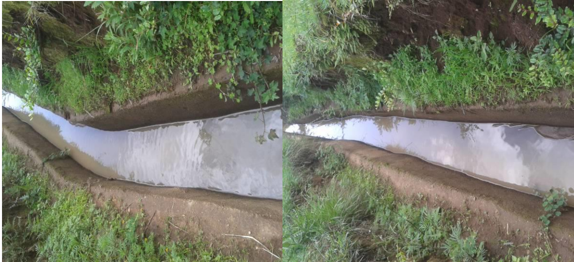
Figure 3.3 Lined Canal of the Scheme
