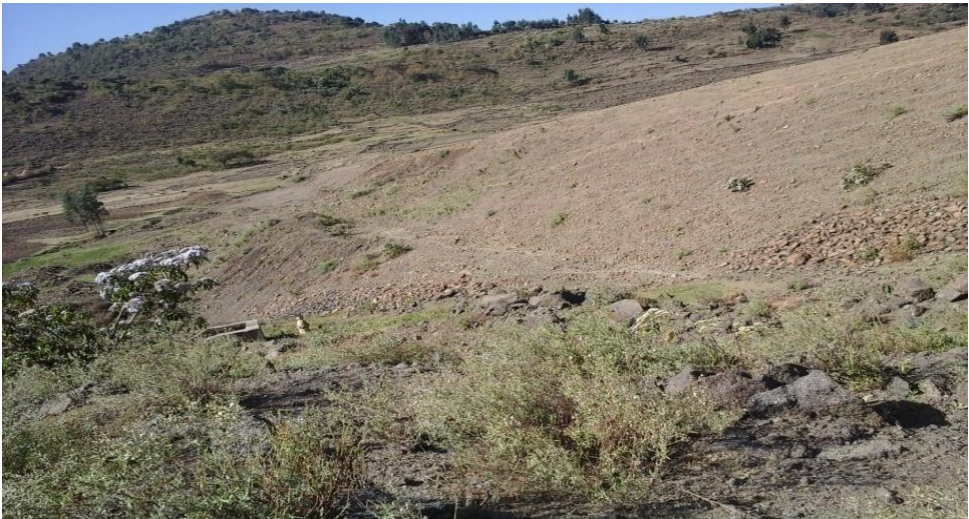
Figure 14 Downstream face of GMED
