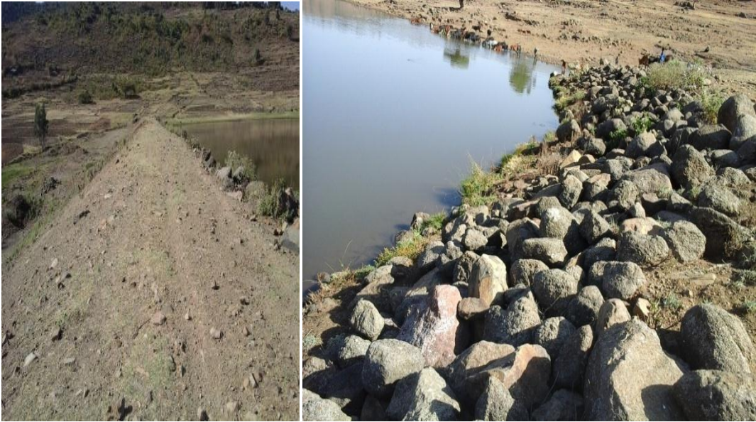
Figure 13 GMED crest and upstream riprap
