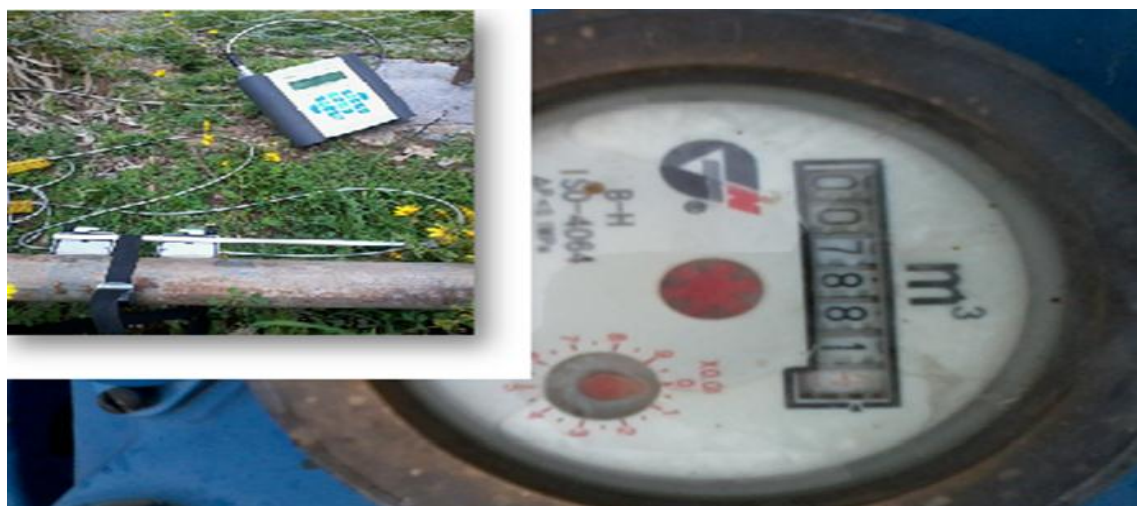
Figure 3.2 Photo during flow measurement by Ultrasonic and Mechanical flow meter
