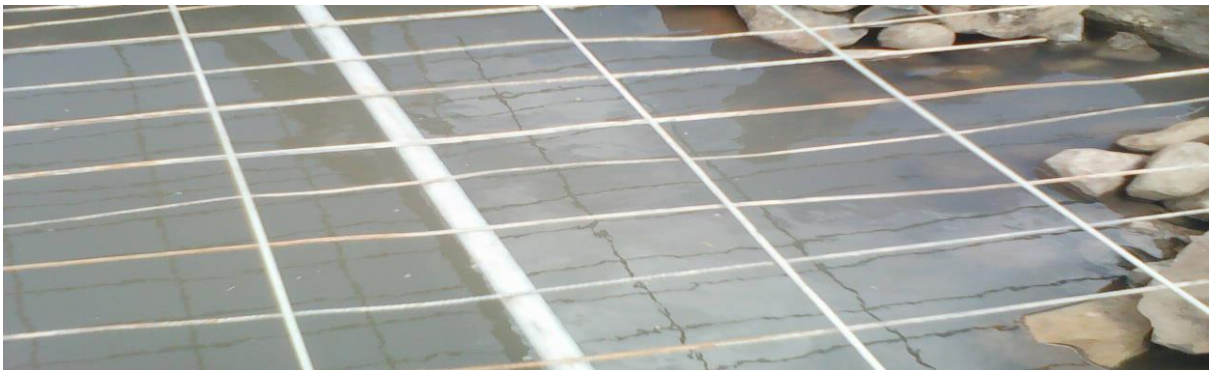
Figure 4. 11 partially covered spring box during construction
