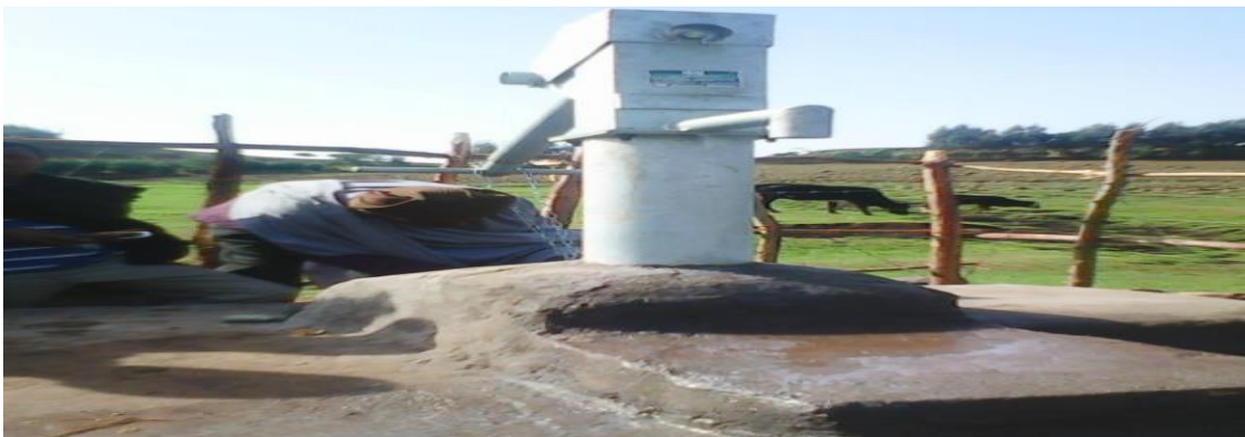
Figure 4. 16 A hand dug well after construction
