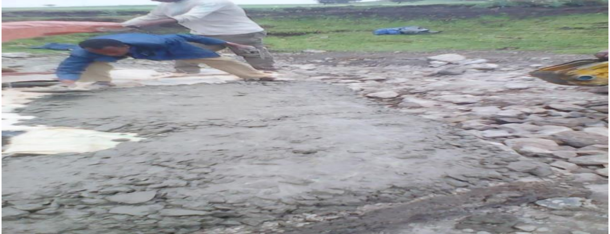
Figure 4. 12 A spring box fully covered by reinforced cement concrete during construction
