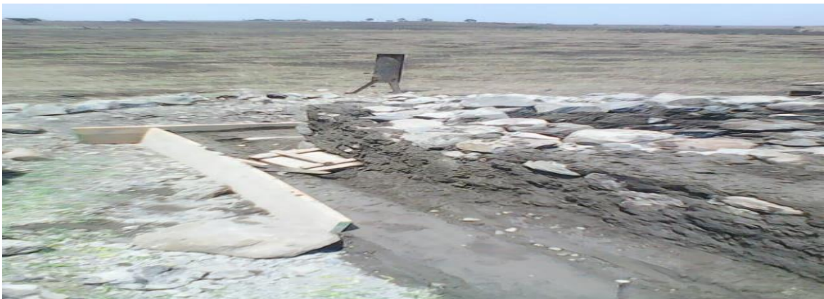
Figure 4. 15 A hand dug well during construction
