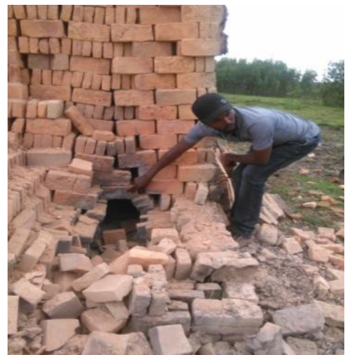
Photo-8 over burned clay brick kilns
