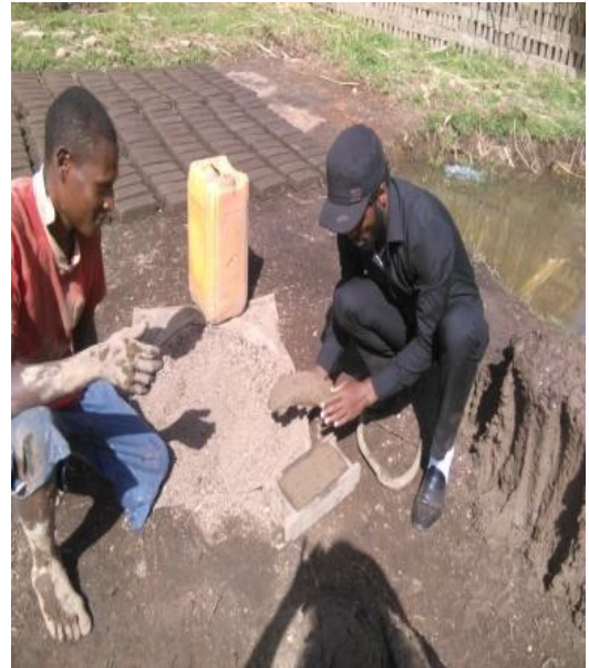
Photo-14 Wood molding of Brick
