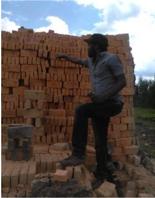
Photo-1 Inspection of fired Bricks in production kiln
