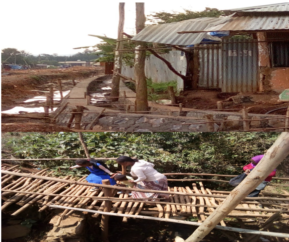
Figure 4.1 Yetebaberut-Wuhafisash and Dippo-Firustale road project
