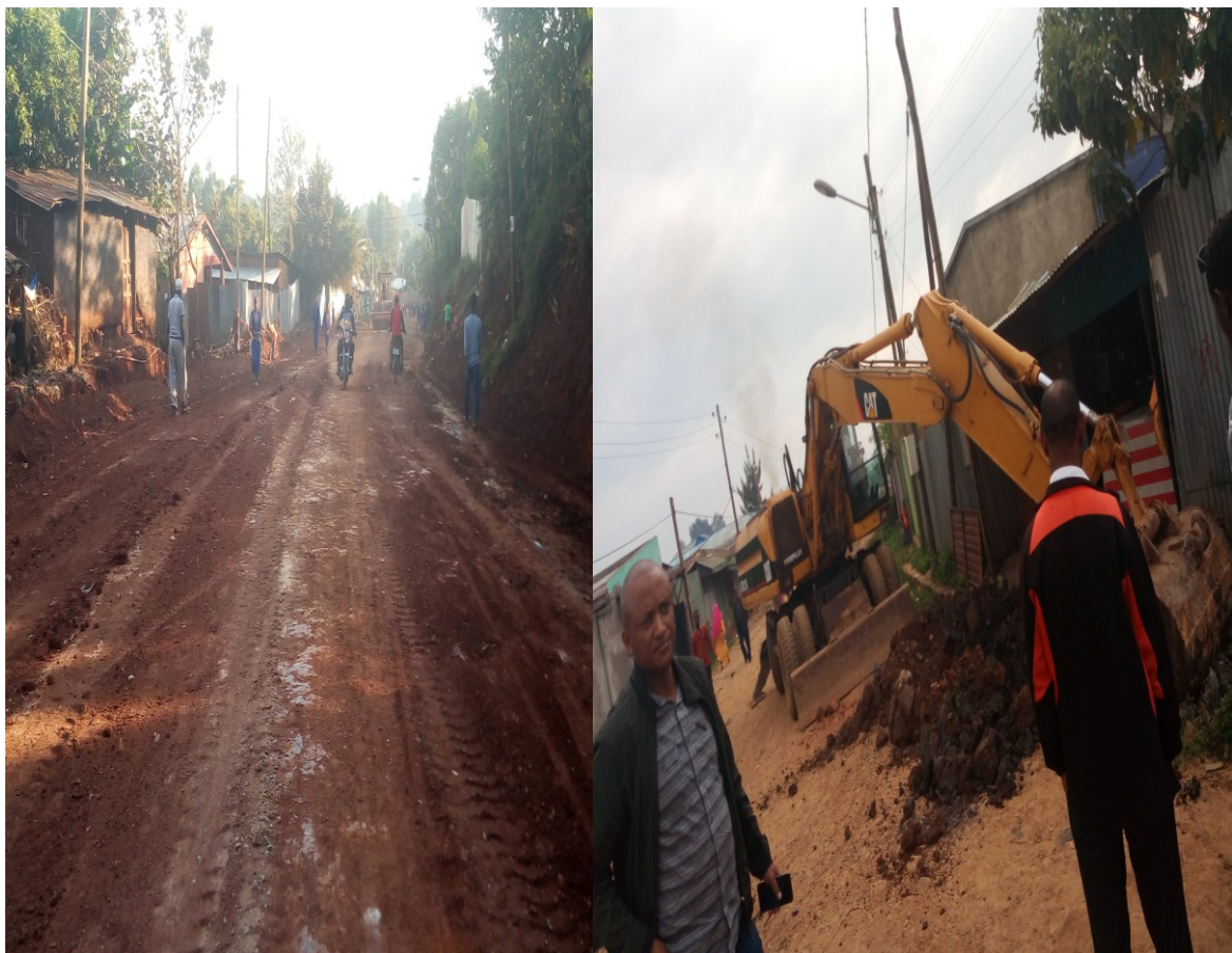
Figure 4.2 Compacted earth road project at different Kebeles.
