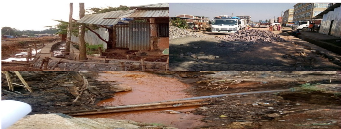
Figure 4.111 Right of way problem and high traffic on the site.
