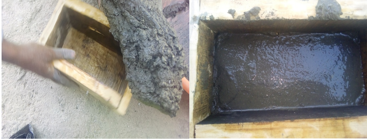
Figure 3.10: Casting the mixed material in mould (16/3/2021)
