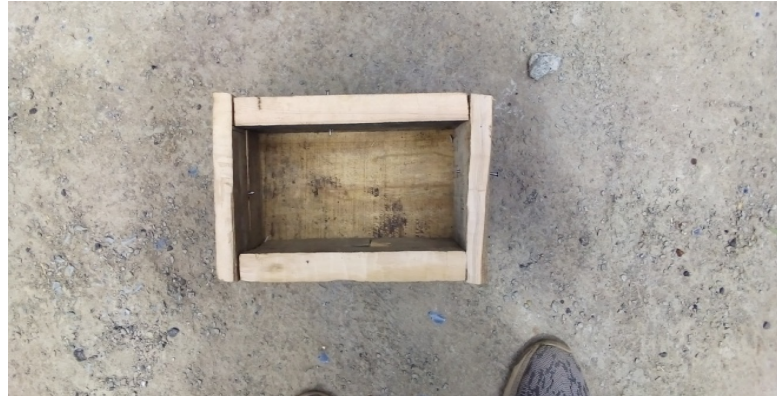
Figure 3.5: Mould preparation in the carpentry shop (3/12/2021)
