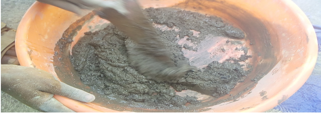
Mixing of ingredient of plastic fly ash bricks (photo taken by me)
