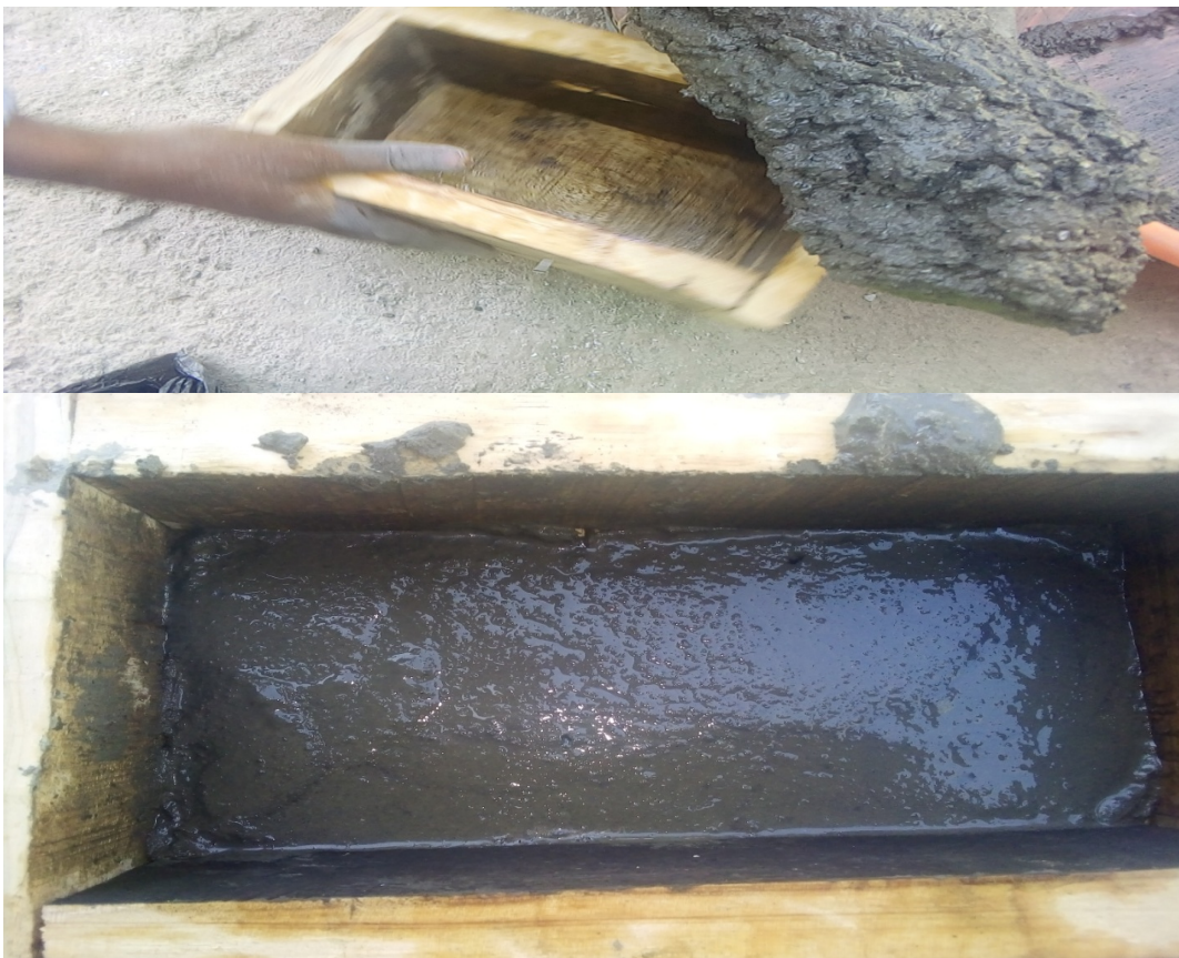
Casting and Moulding of bricks (photo taken by Belete Asegdew)
