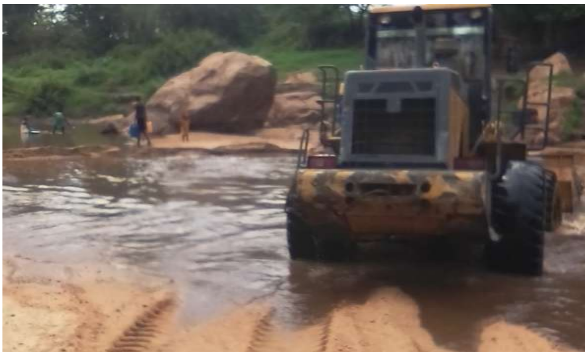
Annexes Figure 16: Front loader extracting river sand
