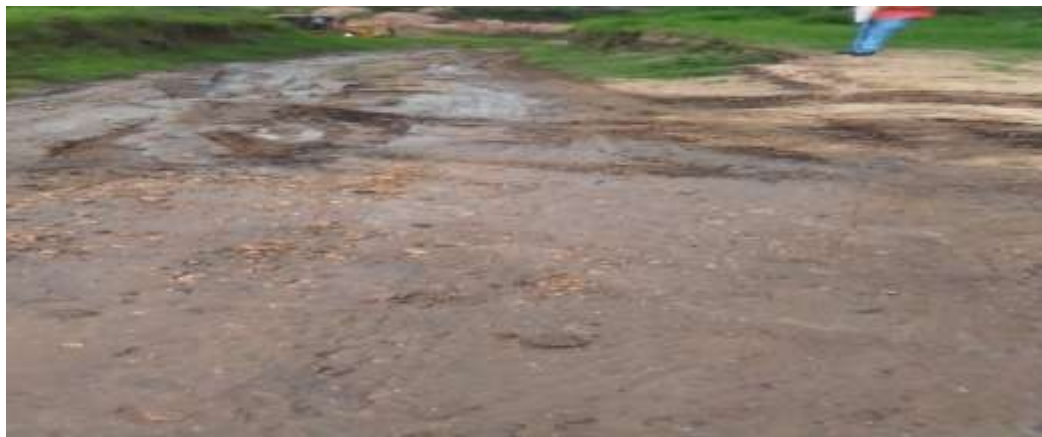
Figure 4. 14: Access routes and stockpiling on river bed
