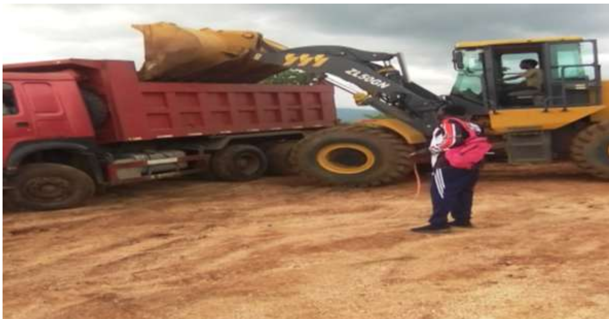
Annexes Figure 6: Front end loader loading Sino-trucks from sampled point site B
