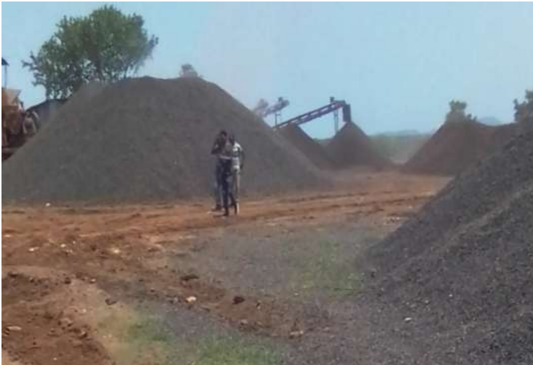
Annexes Figure 14: grinded gravel site machine
