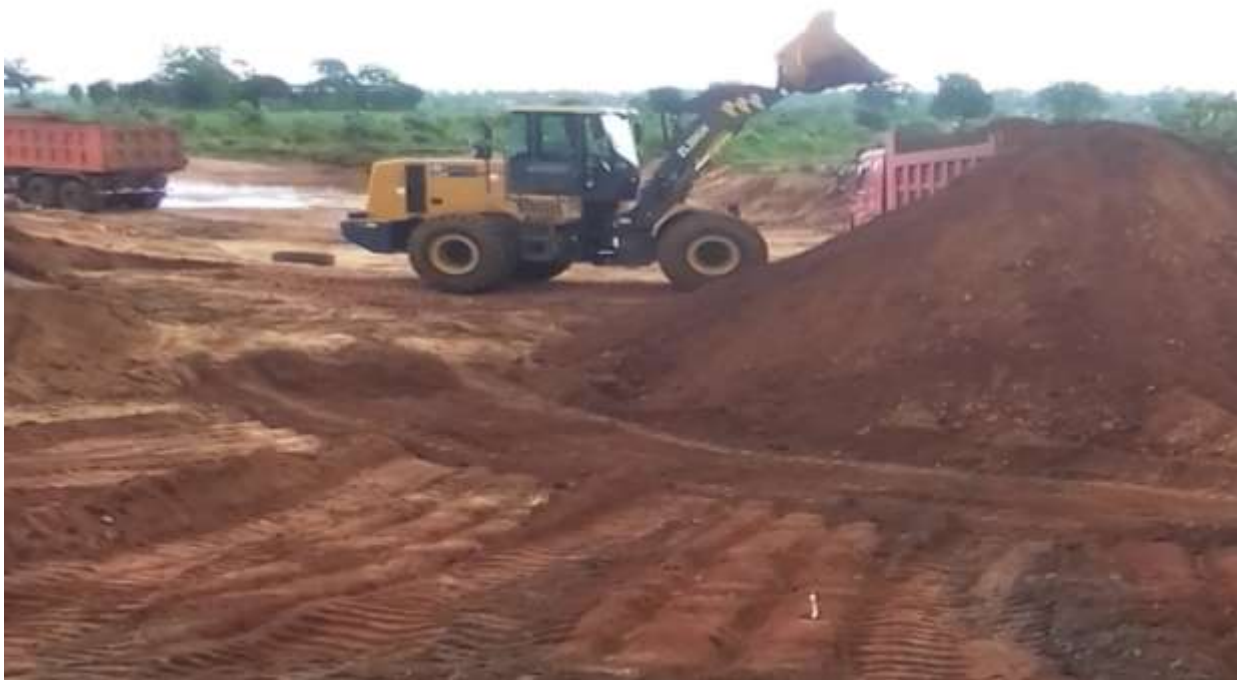
Annexes Figure 15: Extraction soil component site
