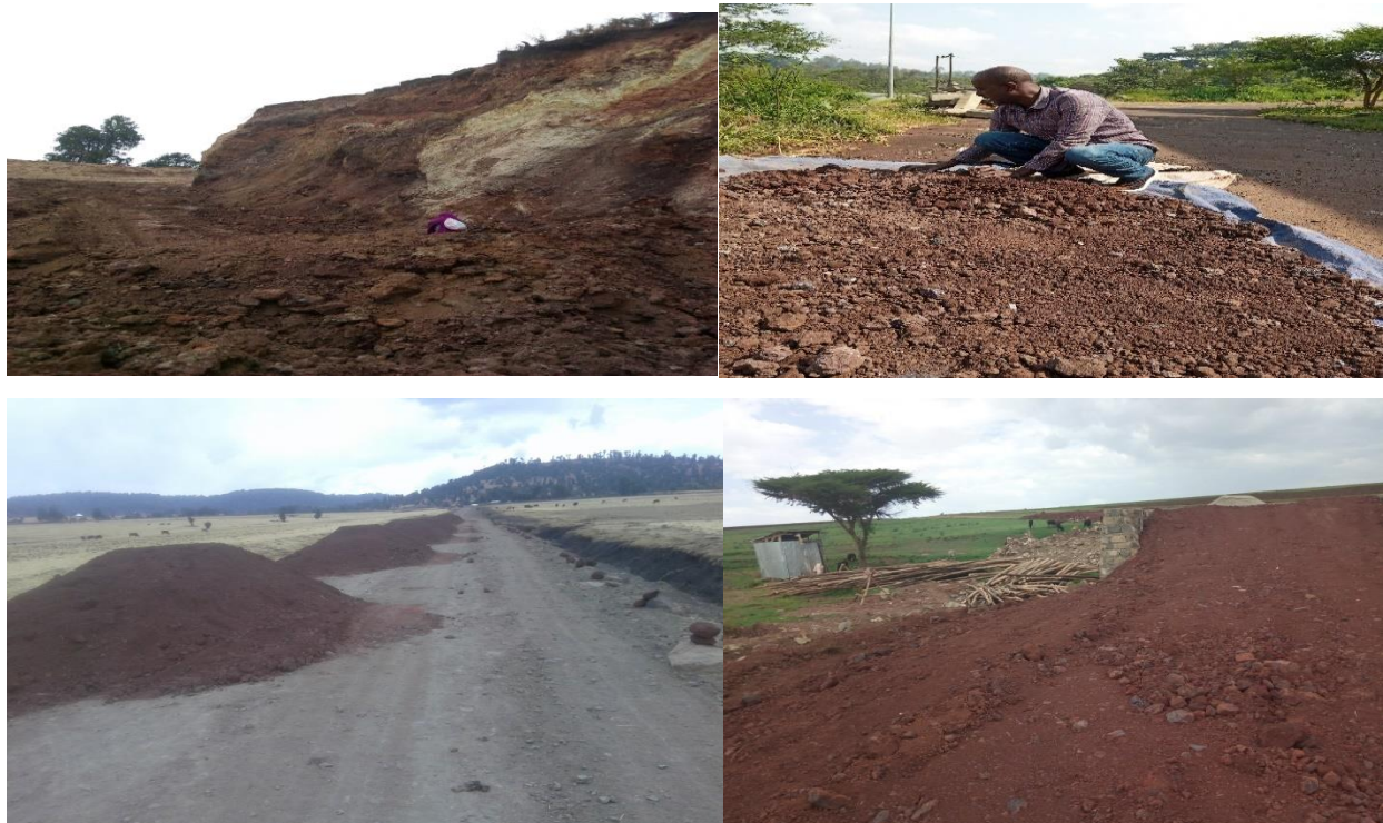
Figure 3-2: Photo shows Cinder Graveling Road surfacing (July 06, 2021, Captured by Getachew)
