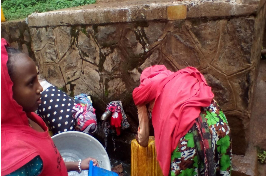
Figure 3: Dawe qäbälé Water Reservoir Built in 1990 by NGO
