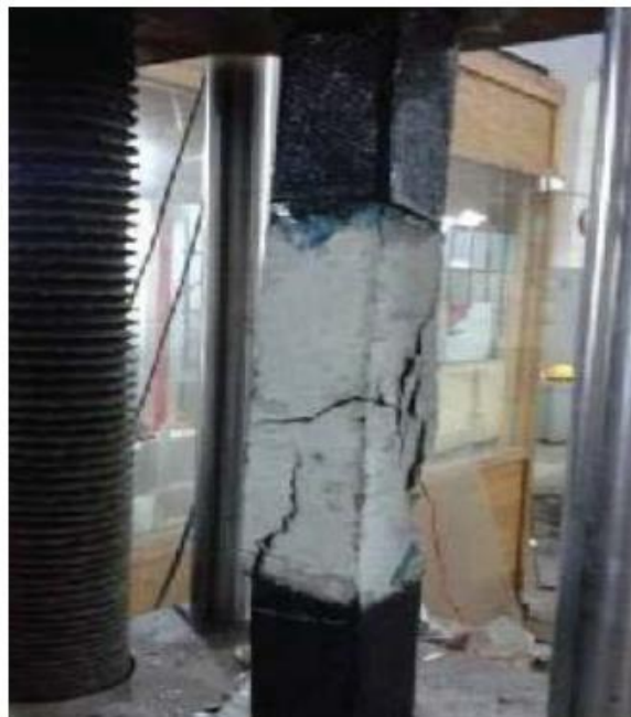
Figure 3.19 Failure mode of a column from experimental study (Rahman, et al., 2016)
