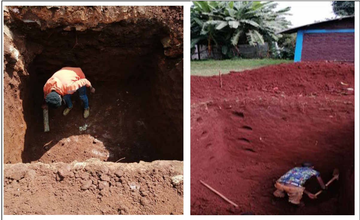
Figure 1: An over view of test pits while soil sample extracted. (Photo captured by Bilisumma L.)
