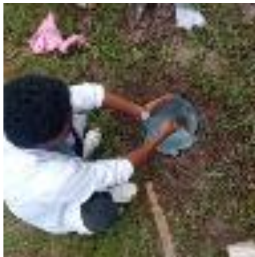
Figure 6. covering pool by plastic
