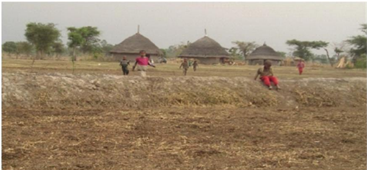
Figure 4.18 Flood protection structure on flat area of Shashogo, in Suta Kebele (source capturing photo from site observation 6/ 24//2020 at 10:45AM).
