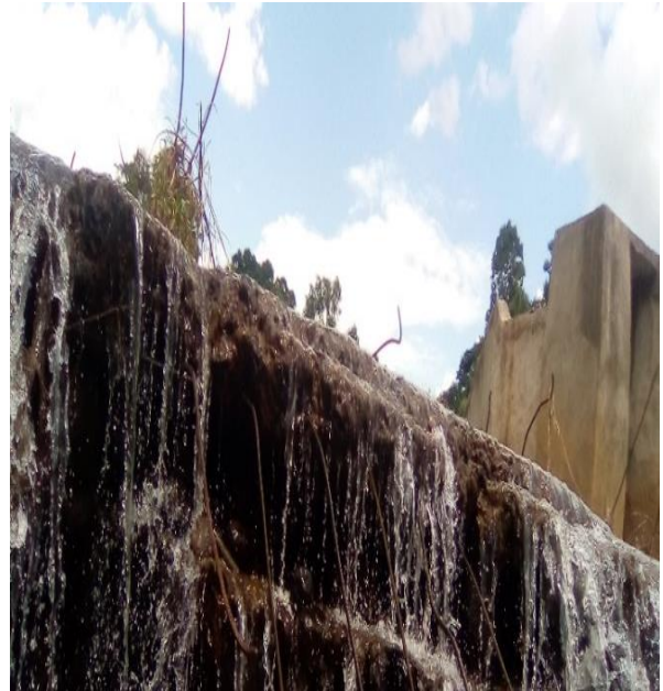
Figure 4. 11:- Effect of improper construction of impervious floor of Offiya weir.
