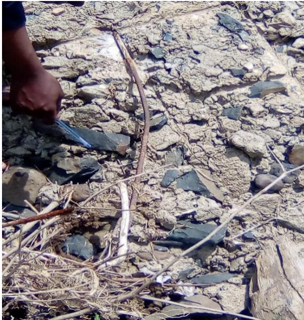
Figure 4. 11:- Effect of improper construction of impervious floor of Offiya weir.
