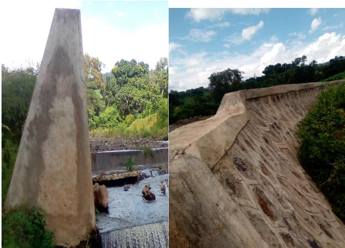
Figure 4. 13:- Offiya retaining wall
