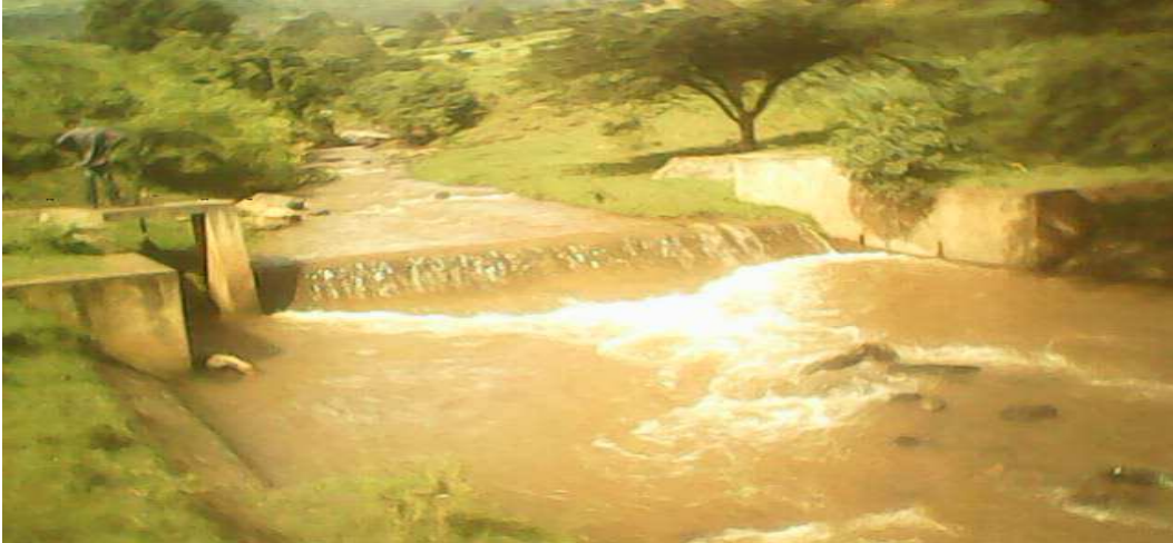
Figure 4.2: Diversion weirs Head Regulator
