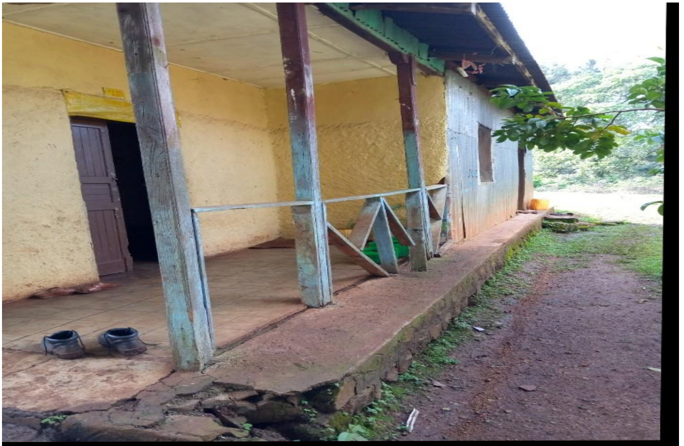
Figure 5: Lej Abata Mulat’s Temporary Residence at his former Dooraa coffee plantation
