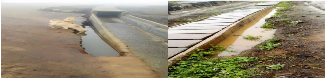
Figure 4. 14 Ponding at sides of U-ditch at Gessa (By: Mengistu Bayu, 21th April, 2021)
