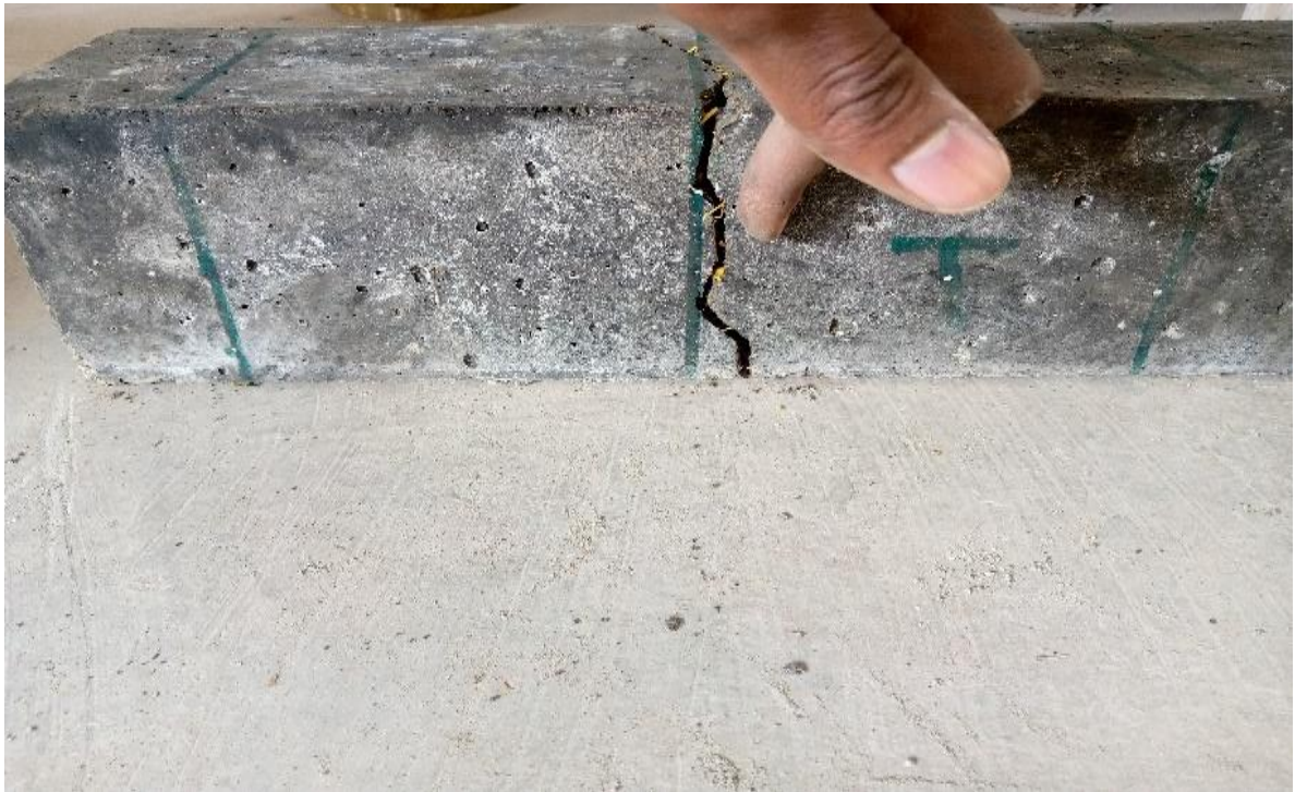
Figure 8. Position of flexural beam failure line.
