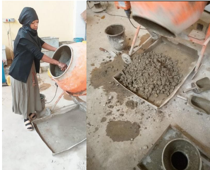
Figure 3.7: Mixing of concrete ingredients
