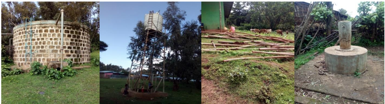
Figure 4: Serviceless reservoirs, pipes and public taps due to design problems
