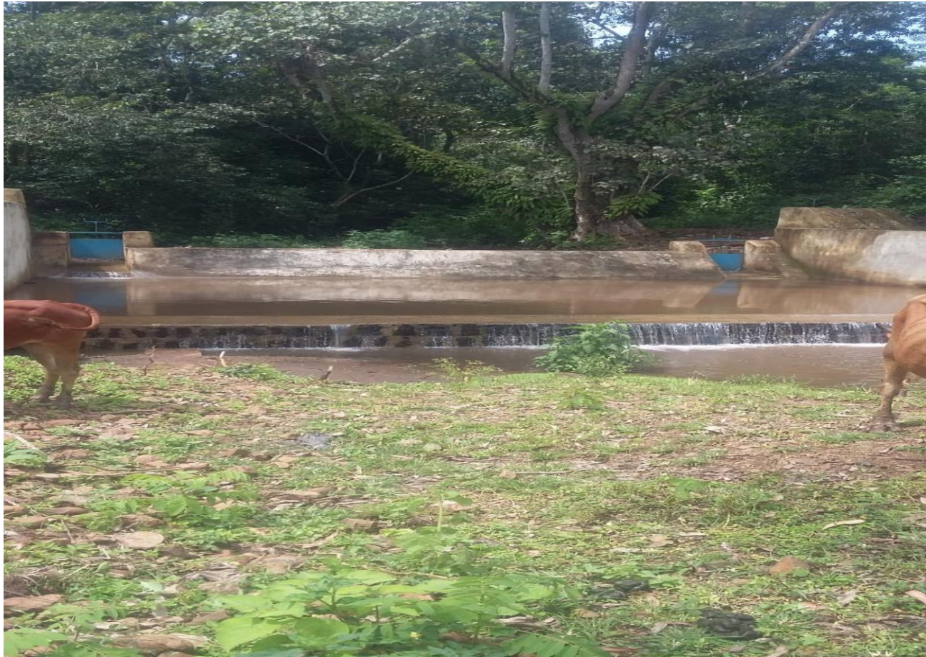
Figure 8: The Hamuma irrigation dam built by SLM; picture by the researcher, Hamuma,(2021)
