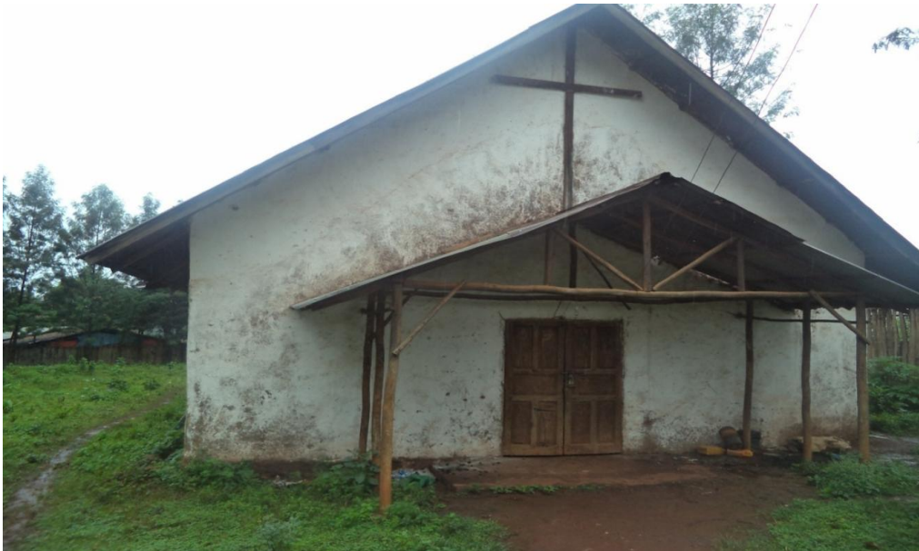
Figure 8: Beghi MYC which is closed by the Dërgand it gave service from 1986-89
