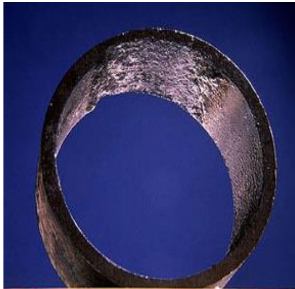
Figure 1: Corrosion of boiler tube and its failure[4].
