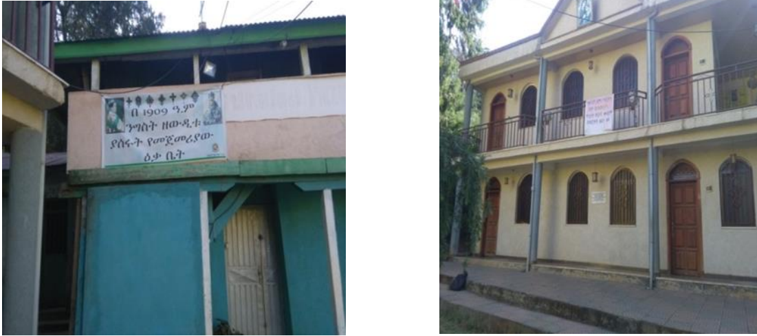
Fig.11. The first Eqa bet of Empress Zewditu (1916) and the new museum buildings.
