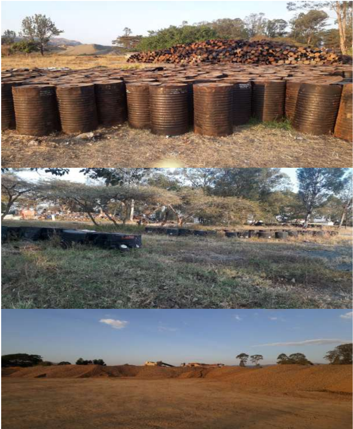
2. Photos during physical observation of construction site
