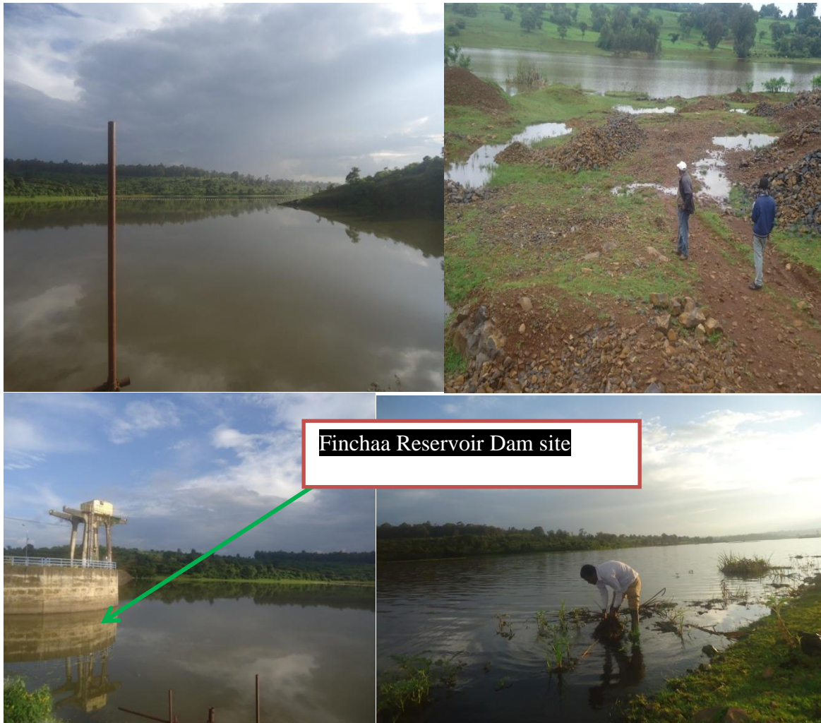
Figure 3. 5 Reservoir area of Finchaa’a watershed (image taken during Field visit).
