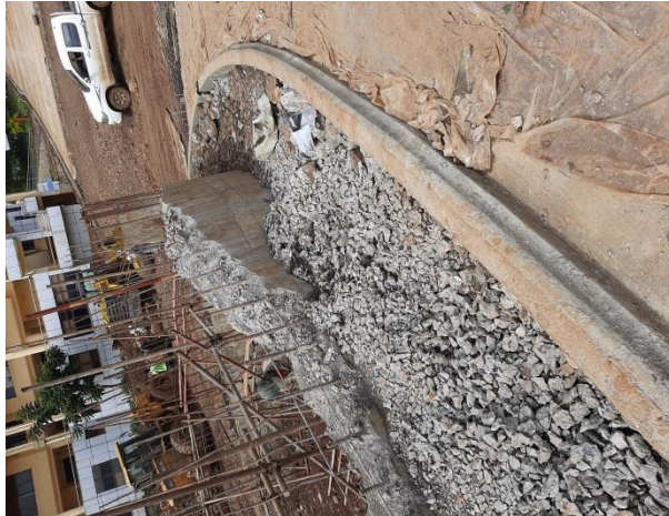
17/7/20, Captured by Kinfe.G/G Demolished concrete waste site
