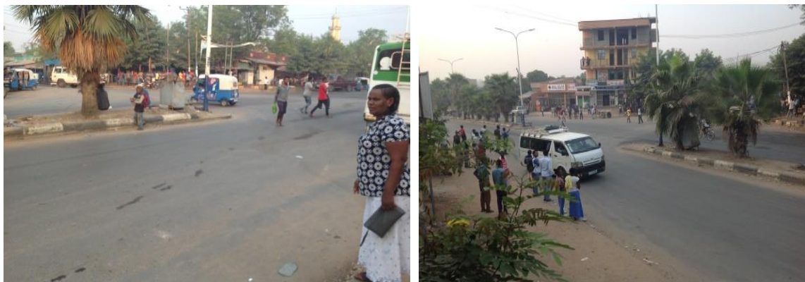
Figure 4.15: Lack of curb cut and curb ramp to enhance pedestrian crossing
