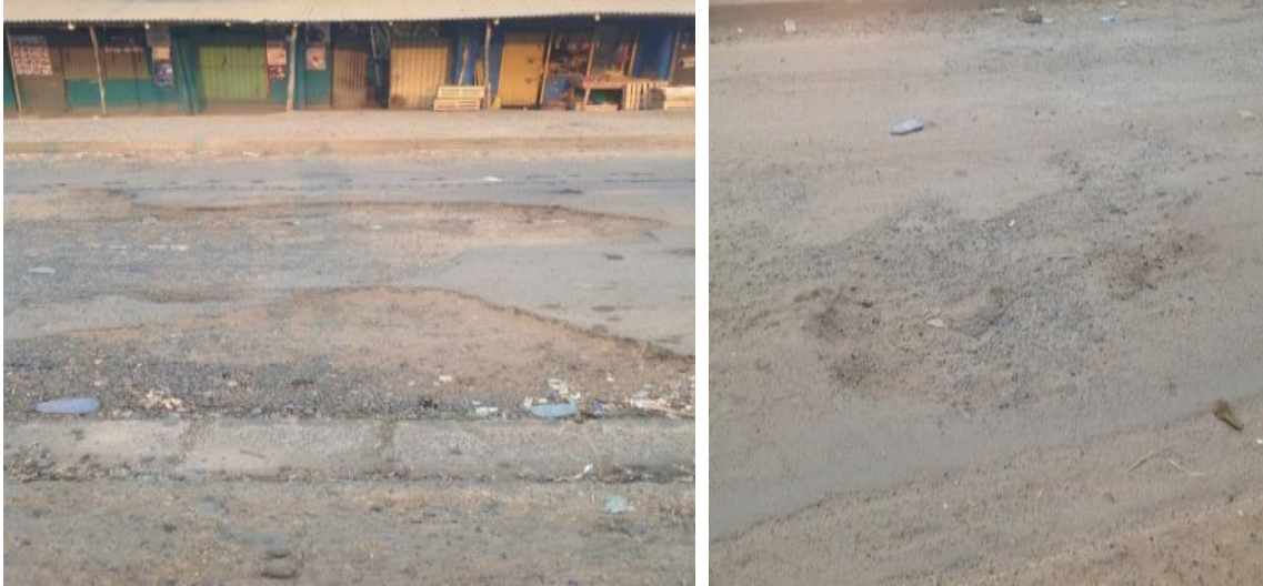
Figure 4.10: Poor crosswalk surface condition and lack of accessible curb ramp and lack of zebra crosswalk marking
