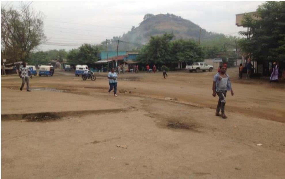
Figure 4.13: Poor crosswalk surface condition, lack of accessible curb ramp and no zebra crossing marking
