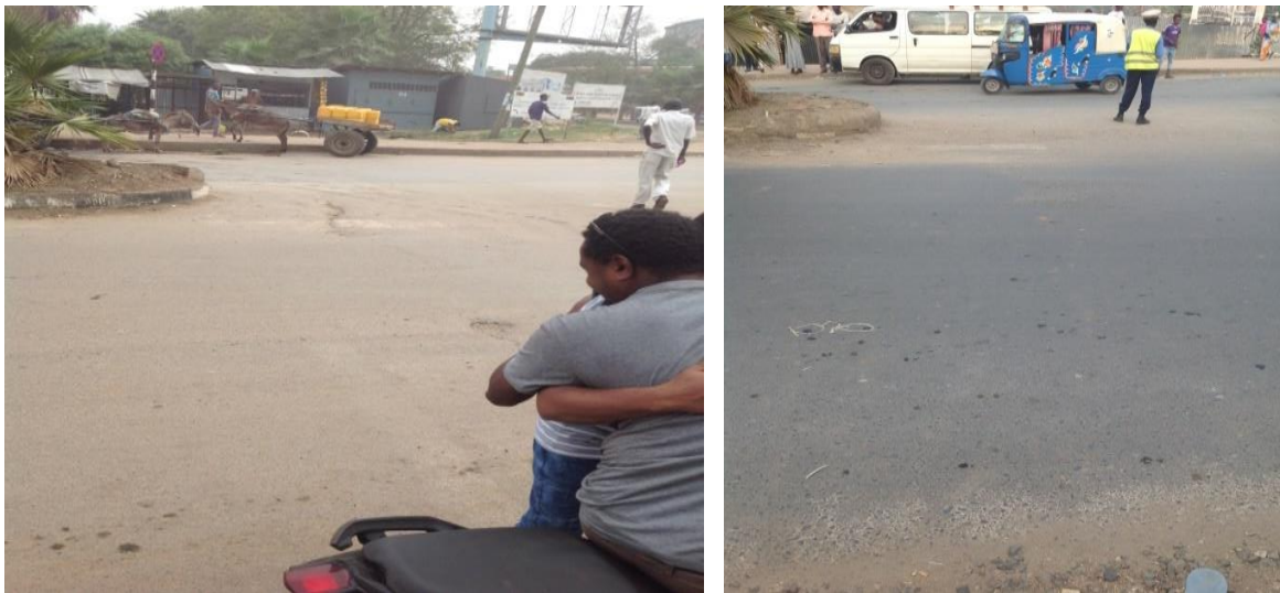
Figure 4.22: Lack of accessible curb ramp on either side of the crosswalk and invisible crosswalk marking
