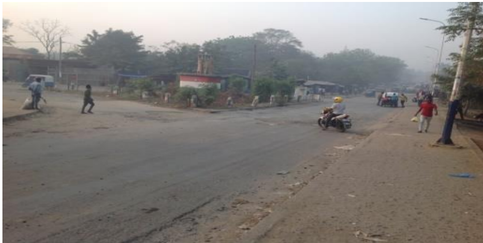
Figure 4.10: Poor crosswalk surface condition and lack of accessible curb ramp and lack of zebra crosswalk marking
