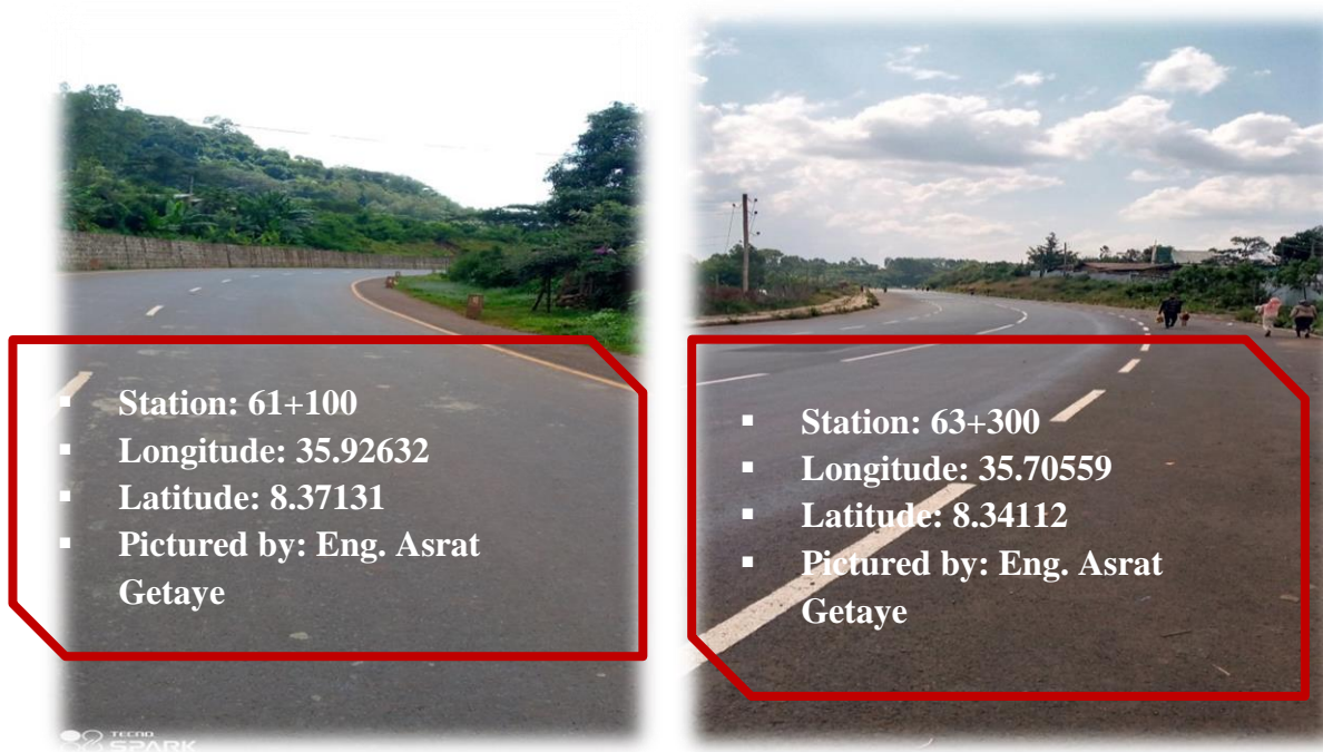
Figure 4.2: Selected normal road sections along Bedele – Metu road upgrading project
