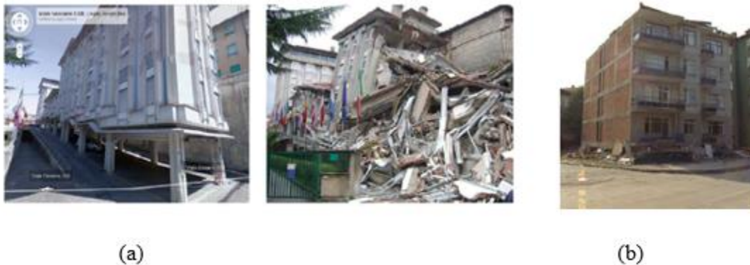
Figure 2.1 Building failures during earthquake (a) L'Aquila 2009, (b) Izmit 1999 [3]
