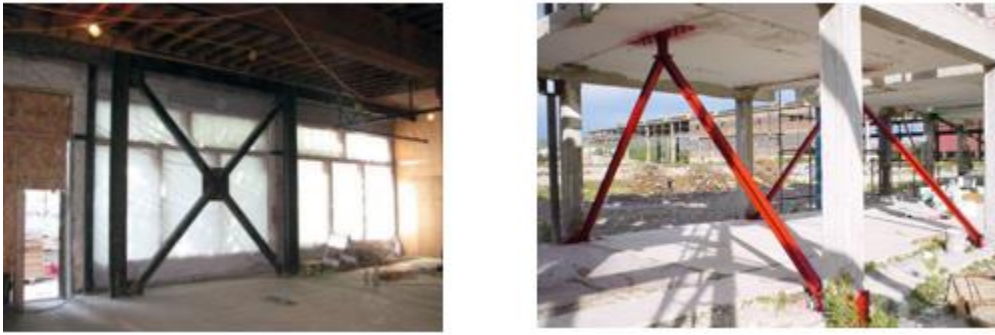
Figure 2.4 Application of Concentric bracings for retrofitting [9]
