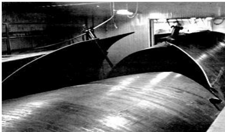
Figure 1.1 Pressure vessel welded joint failure (Atreya and Engineering, 2017)
