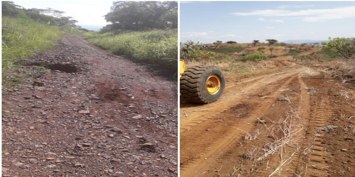
Figure 1.21 URRAP Road under reconstruction due to delay
