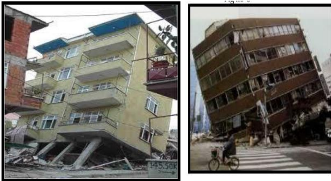
Figure 2. 7: Failure of structure due to soft storey effect (GhalimathAG and Hatti MA 2015).
