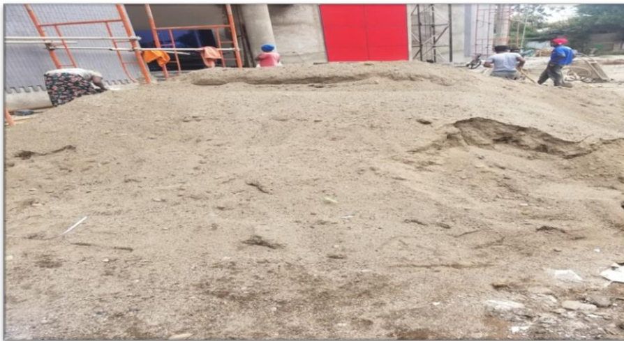
Figure 4.3 Site storage of fine aggregate
