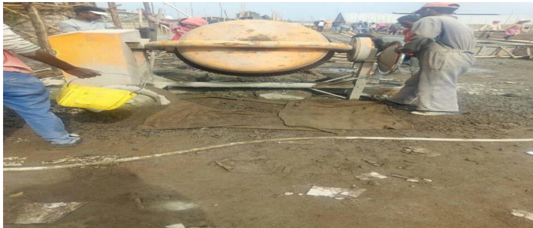
Figure 4.8 Machine mixing of concrete on site
