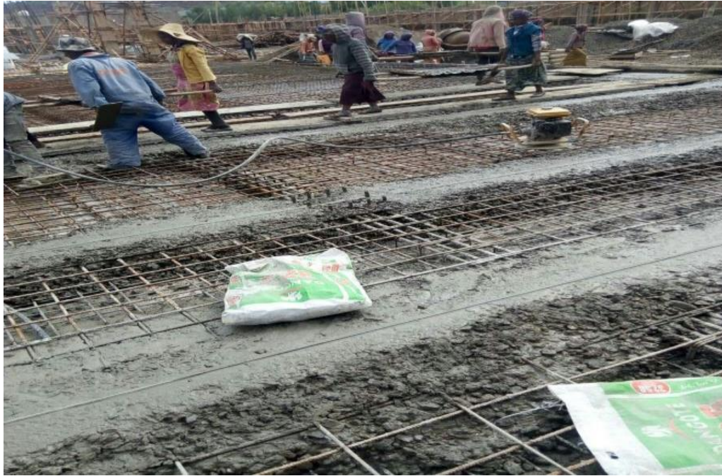
Figure 4.9 Mechanical compaction of concrete by immersion vibratory
