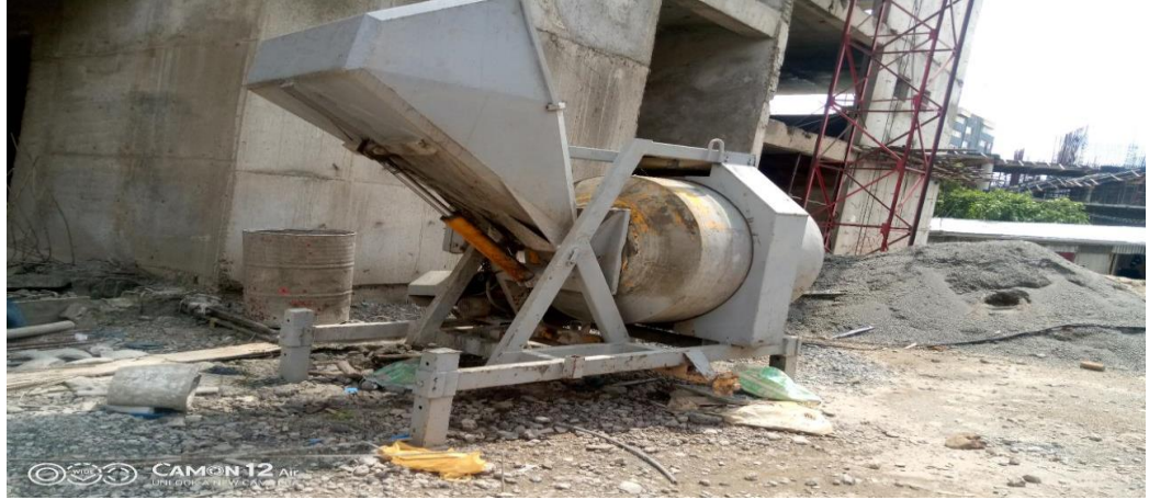
Figure 4.7 Mechanical mixer of 0.36m 3 capacity
