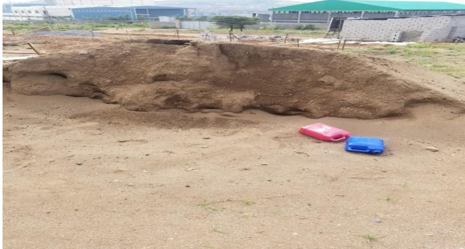
Figure 4.4 Poor quality stockpile of fine aggregate
