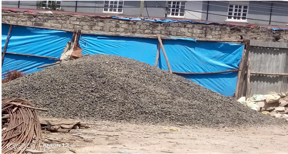
Figure 4.2 Site storage of coarse aggregate
