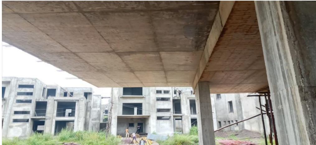
Figure4.5 velvet post tensioning slab with 5m cantilever
