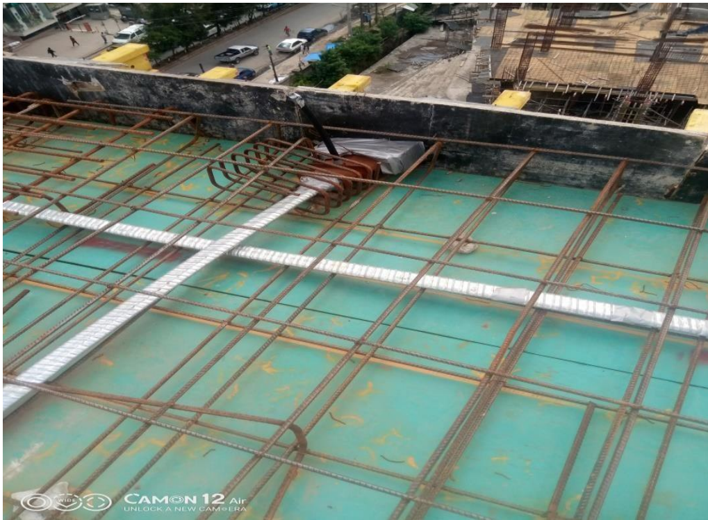
Figure4.24 live end anchorage
