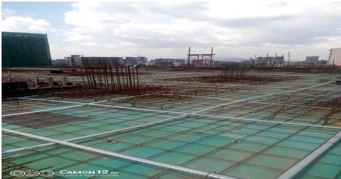
Figure4.3 Joberg post tensioning tendon installation.
