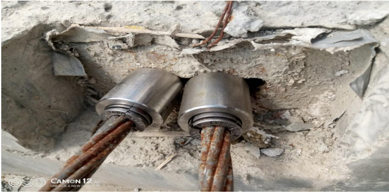
Figure4.13 how to install wedge
