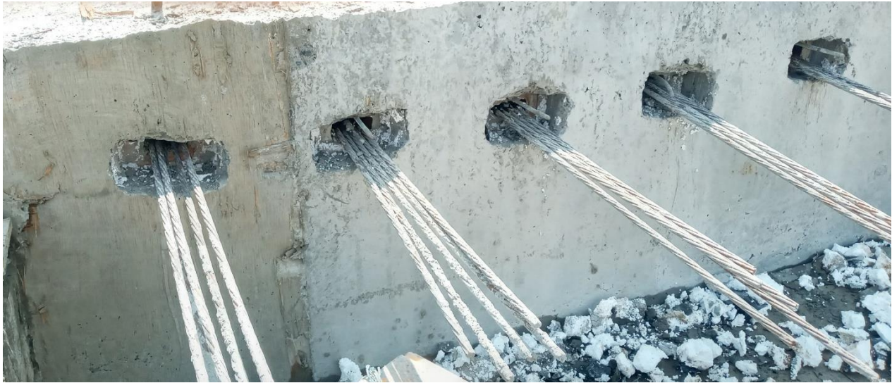
Figure4.26 cutting strand and mortar fill part/stressing whole
