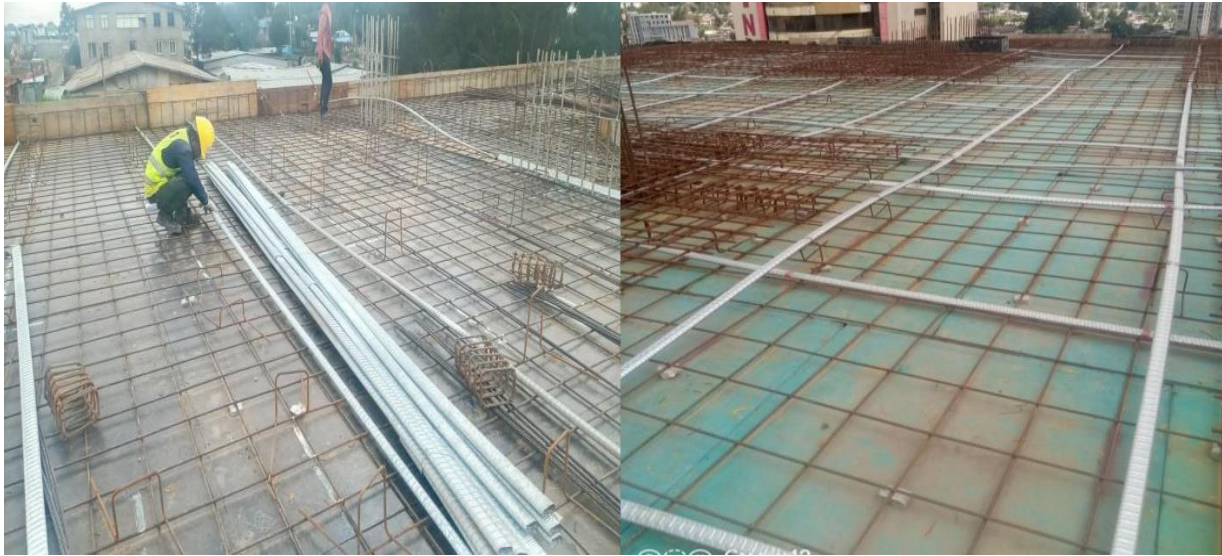
Figure4.11 duct and duct installation
