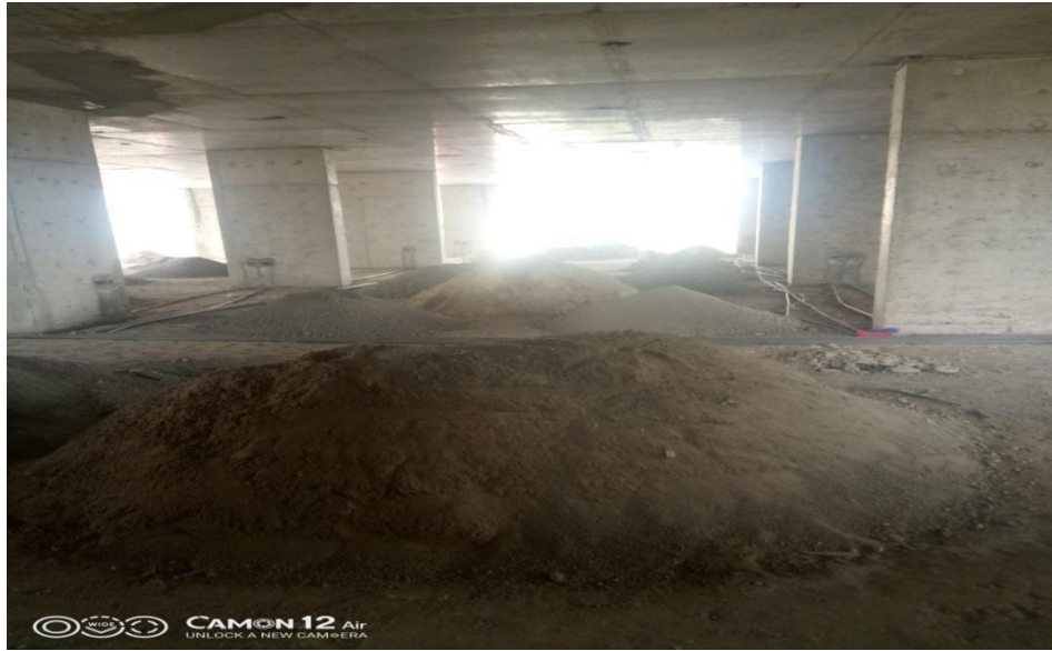
Figure4.2 joberg post tensioning slab all form work removed after 7 days.
