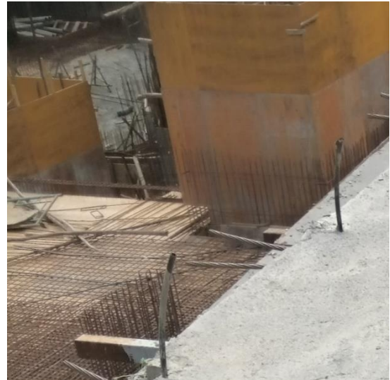
Figure4.27 grouting vent pipe after and before concrete casting
