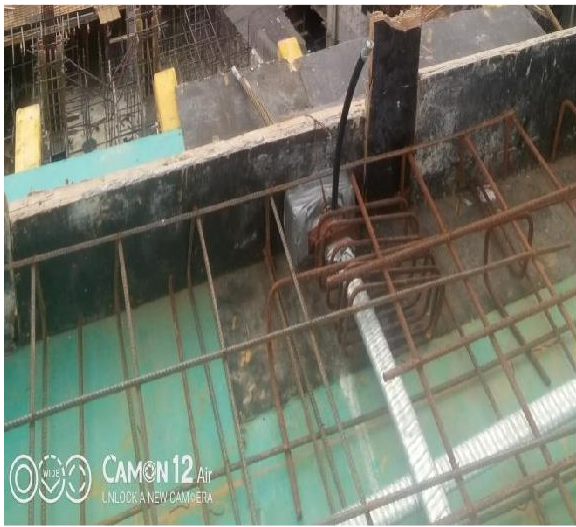
Figure4.27 grouting vent pipe after and before concrete casting
