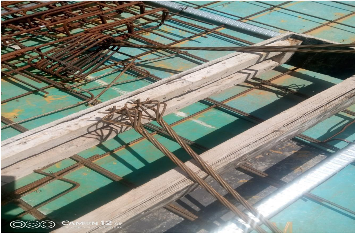
Figure4.25 dead end anchor
