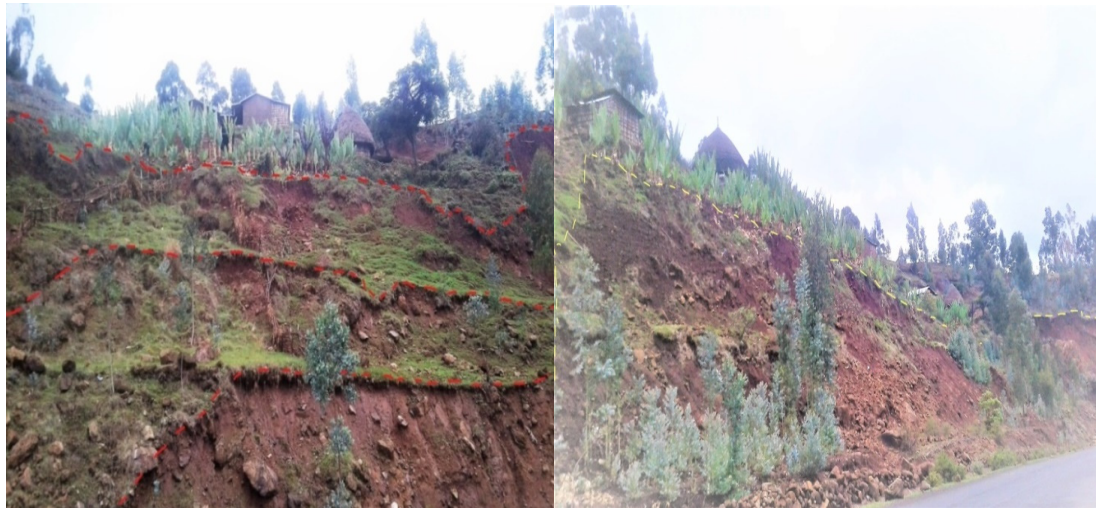
a. Creeping of soil mass causes slope failure.
