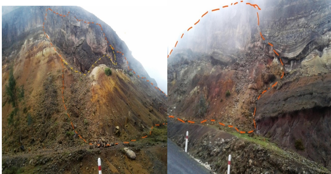
c. Weathered rock along with slope failure
