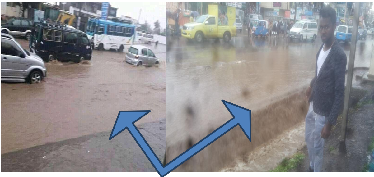
Figure 4.6 inadequate road drainage (over flow) around Kenteri/ Alemgane
