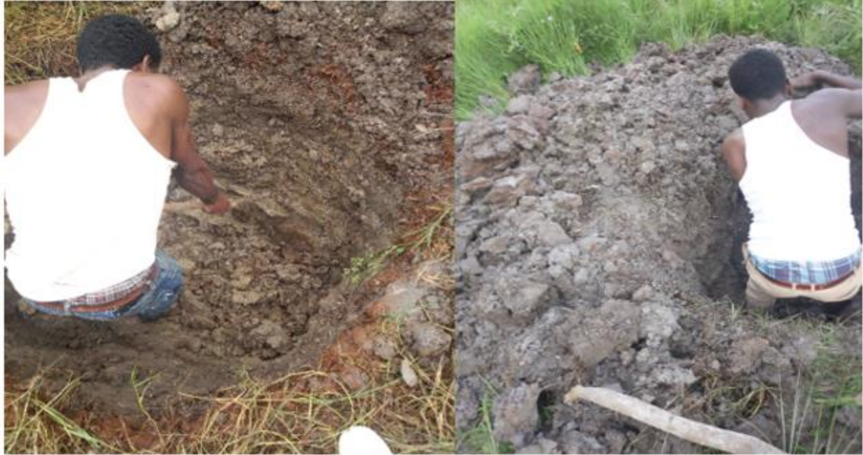
Figure 3.3 Excavated test pits
