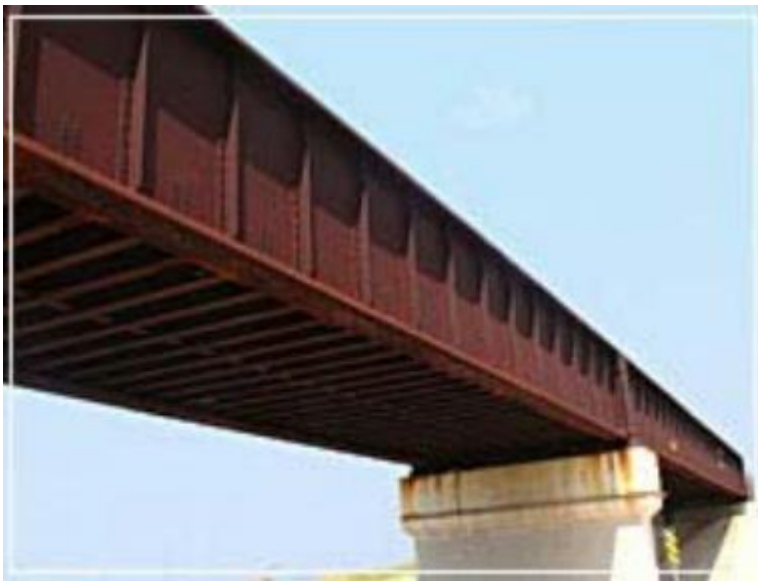
Figure 1-1 plate girder
