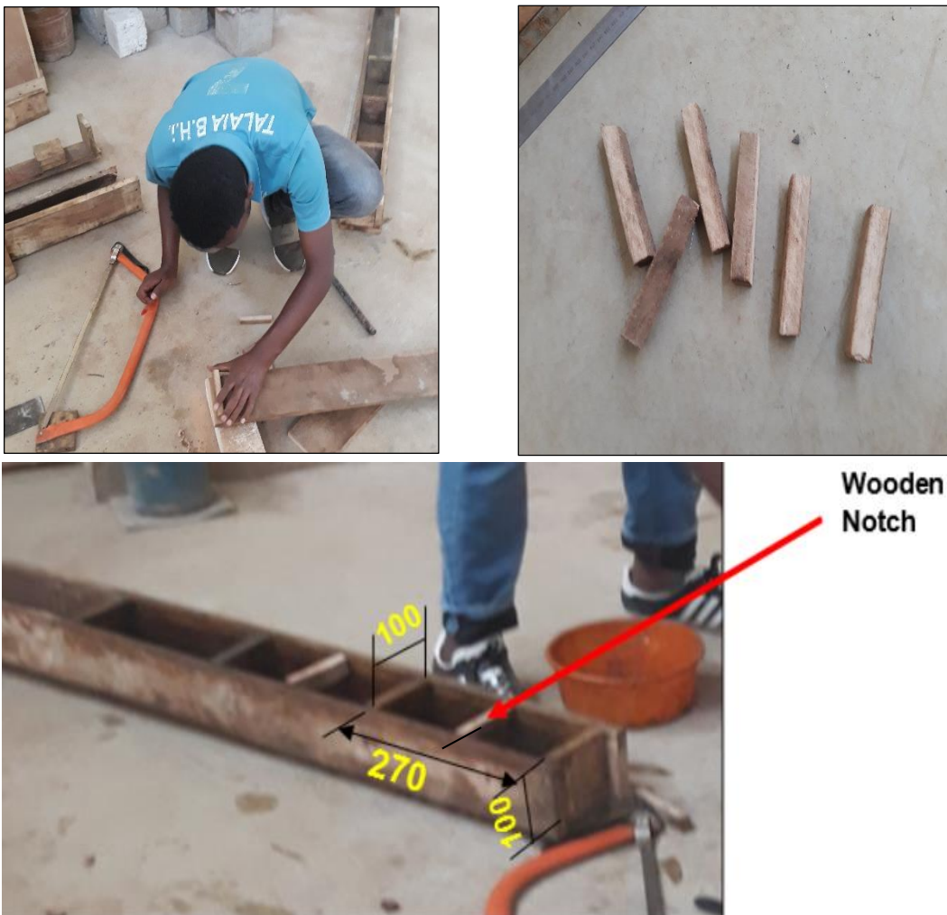
Figure 3-8 Preparation of wooden notches and block dimension
