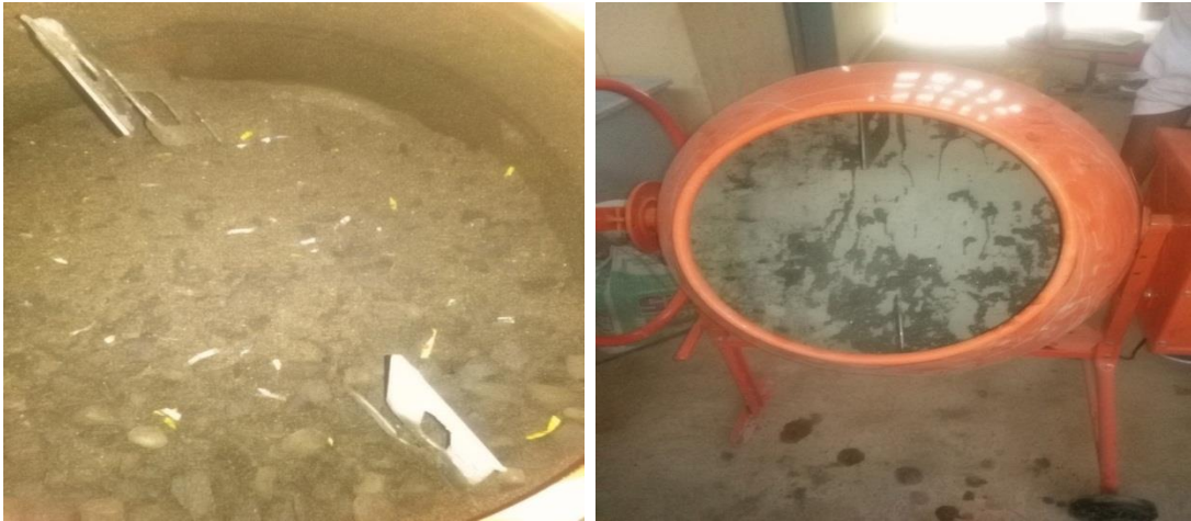
Picture-10: Concrete preparation (mixing of concrete)
