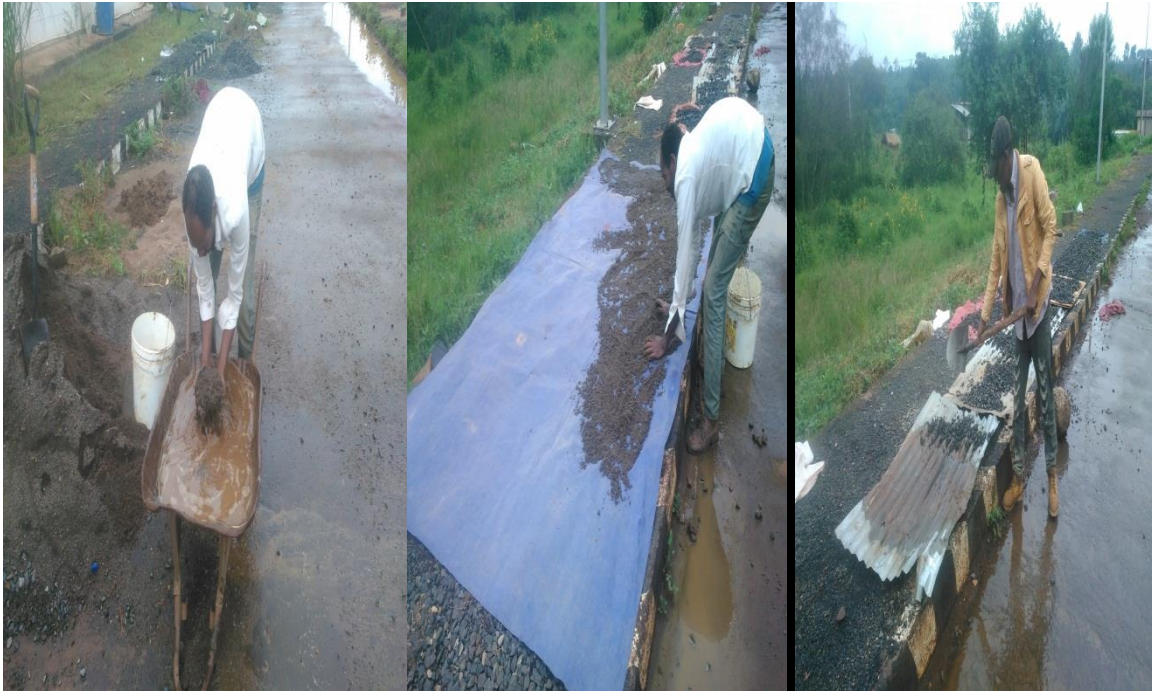
Picture-8: Washing and surface drying of aggregates
