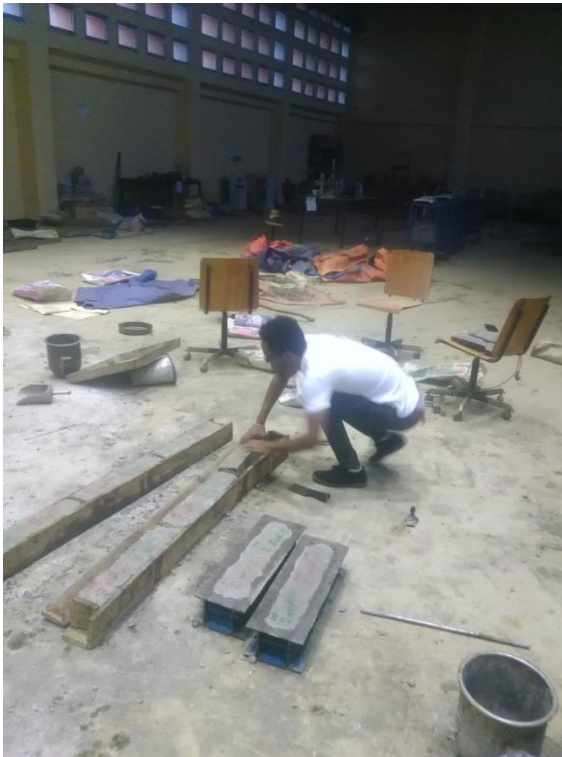
C, Removing of formworks
