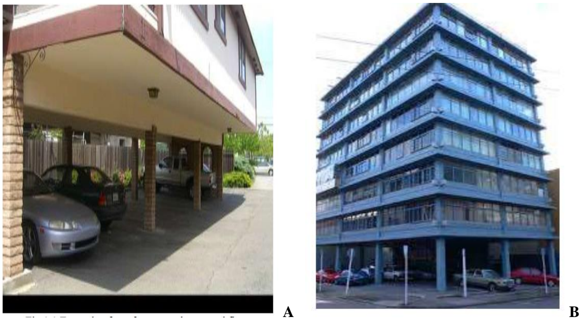
Figure 2. (A) Ground soft storey building & (B) Soft storey in the above level building (Patnala & Ramancharla 2014)
